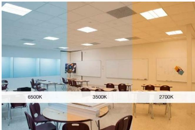
The heart of the NICLS technology is an LED module consisting of separate assemblies of warm-white and cool-white LEDs. Together with sensors and a controller, the NICLS fixtures form a made-in-USA system operated from a user interface that's either mounted in the front of a classroom or accessed
