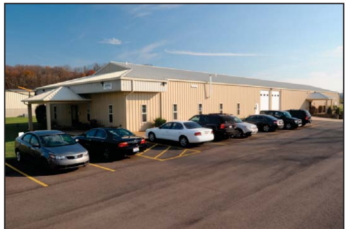
An innovative cool roof installation increased energy efficiency at the Fernald Preserve, Ohio, offsite administrative building.
