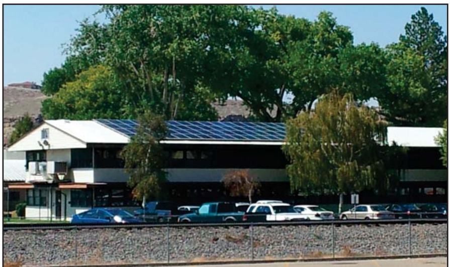
Nearly 90 roof-top solar panels were installed at the Grand Junction, Colorado, site office to lower costs and reduce energy needs.
