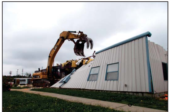
A building is demolished at the Weldon Spring, Missouri, Site.
