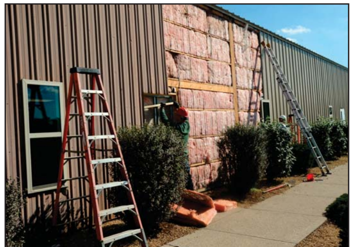
"Cool roof" technology was used on three sides of the offsite administrative building of the Fernald Preserve in Ohio when the old siding was removed and replaced with cool metal similar to that used on the roof.
