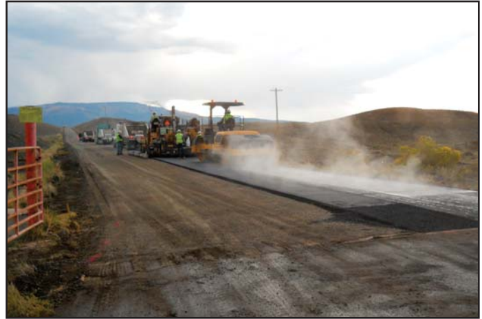
A road is improved at the Grand Junction, Colorado, Disposal Site.
