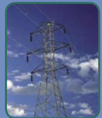
Electric power lines in the Denver metro area
