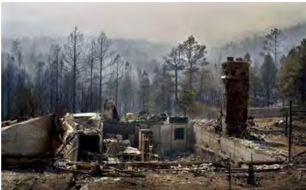
PHOTO 3.1— Burned Residential Unit in Los Alamos Townsite
