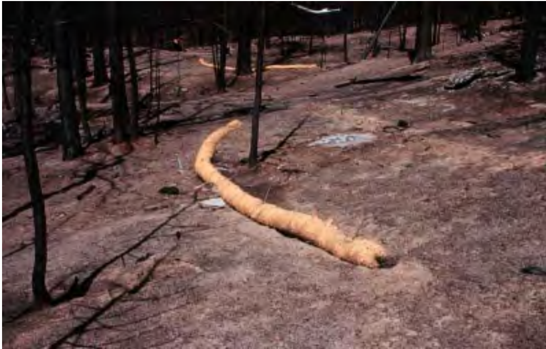
PHOTO 2.12—Straw Wattles in Severely Burned Area
