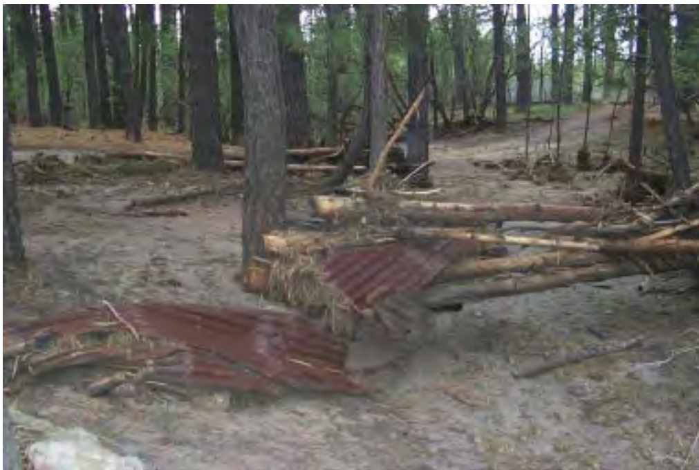
PHOTO 3.6—Anchor Ranch Icehouse after Flooding
