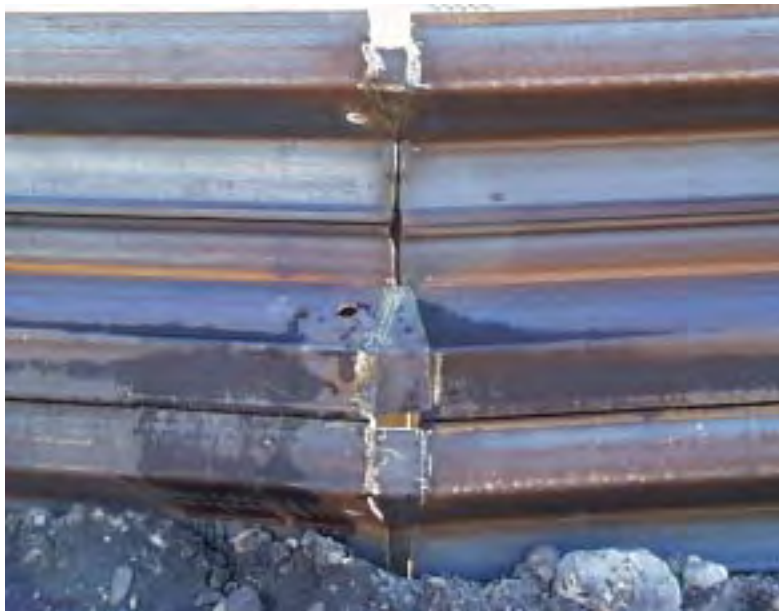
PHOTO 2.21 — Detail of Joined Steel Panel
