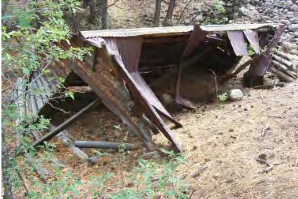
PHOTO 3.5—Anchor Ranch Icehouse before June 28, 2000, Flooding
