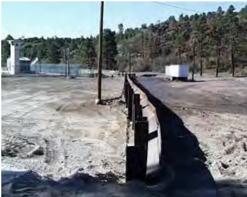
PHOTO 2.20 — Steel Diversion Wall at TA-18 Under Construction
