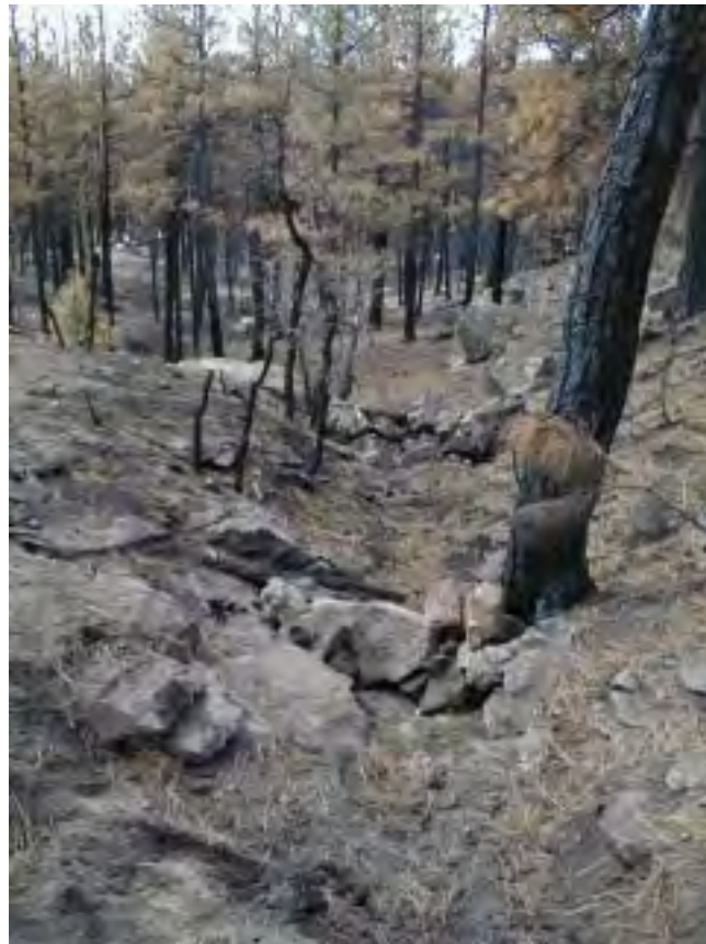
PHOTO 2.11— Rock Check Dam on Burned Slope
