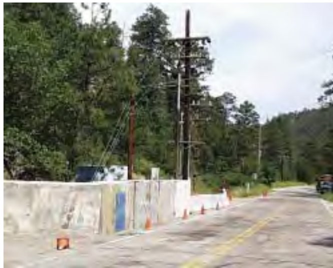
PHOTO 2.13—Storm Water Protection around Utility Pole
