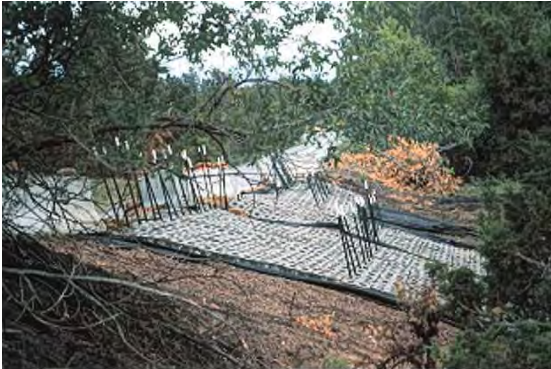
PHOTO 2.18—ACMs Used to Reinforce Road
