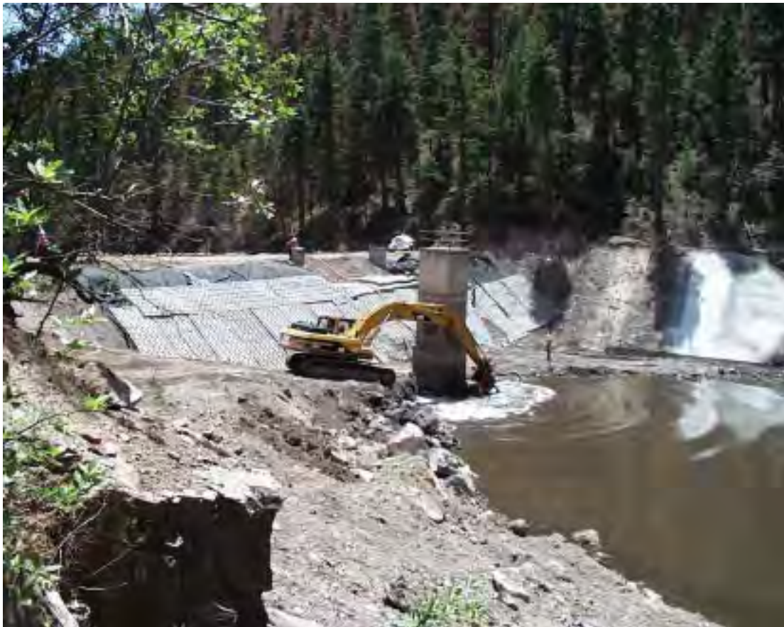
PHOTO 2.15—Reinforcing Los Alamos Reservoir
