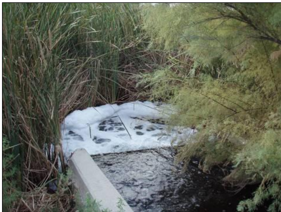
Figure 3.11. Effluent discharge from Gulf Coast Waste Disposal Authority Odessa South Facility into Monahans Draw Impoundment.
