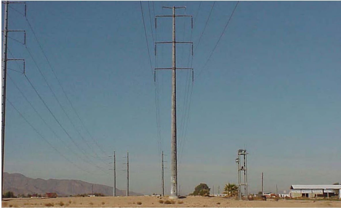
FIGURE 2.2-13 TYPICAL DOUBLE-CIRCUIT 345-kV POLE STRUCTURE
