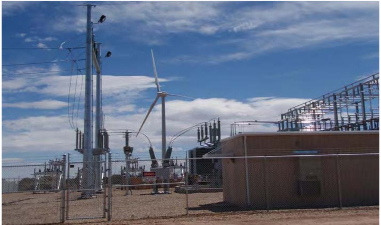
FIGURE 2.2-10 TYPICAL STEP-UP SUBSTATION
