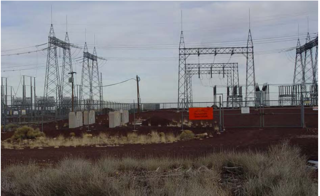
FIGURE 2.2-19 TYPICAL 345-kV SWITCHYARD
