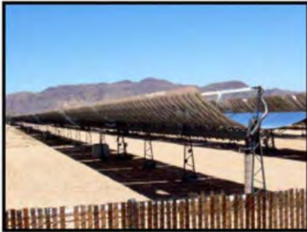
Parabolic trough technology as used in Daggett, CA
