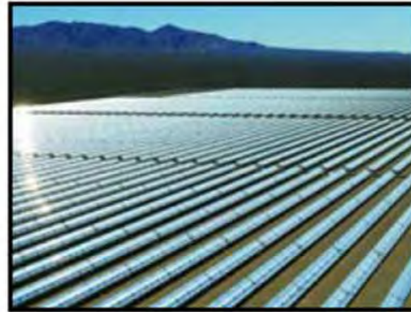
Parabolic trough technology in a 64 MW field (Nevada SolarOne in Boulder City, NV)
