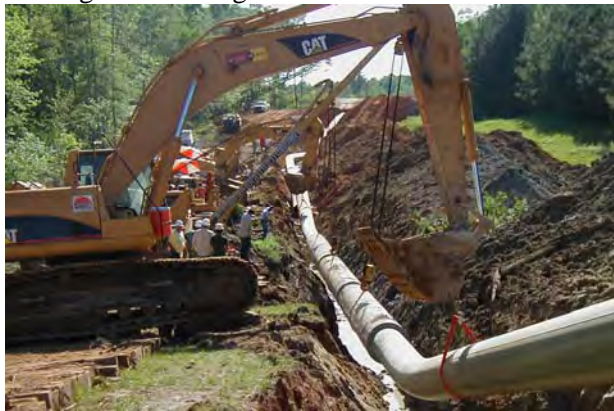
Laying Pipe and Backfilling
