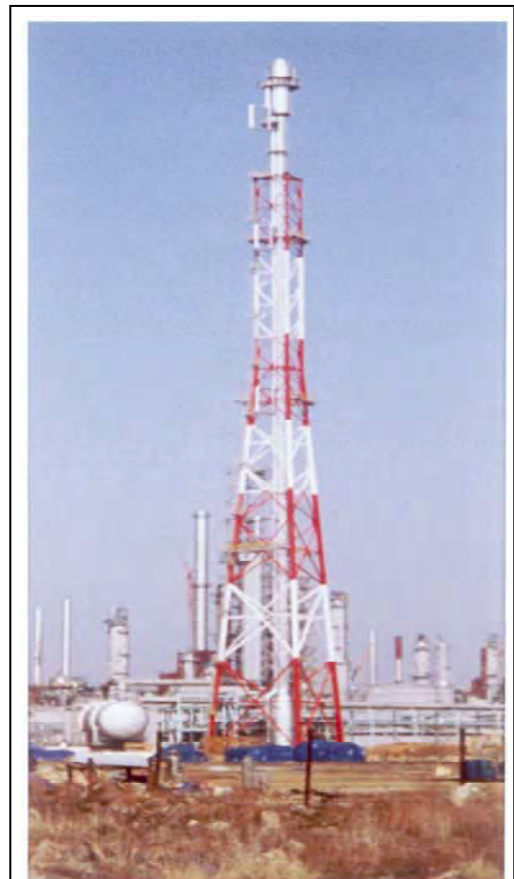
Figure 2.1-9. Typical Flare Derrick with a Single Flare
