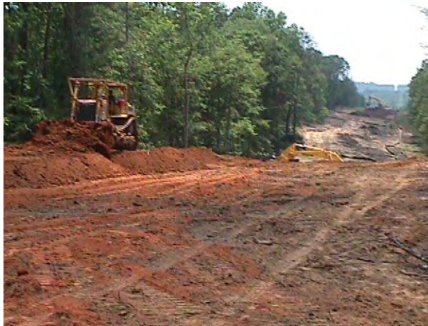
Clearing and Grading
