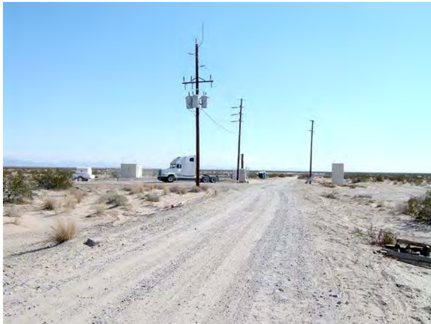
Figure 6. FTHL MA, facing east toward proposed staging area location.
