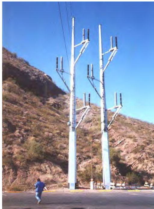
Figure 17. 230 kV extruded dielectric cable riser poles used by Arizona Public Service
