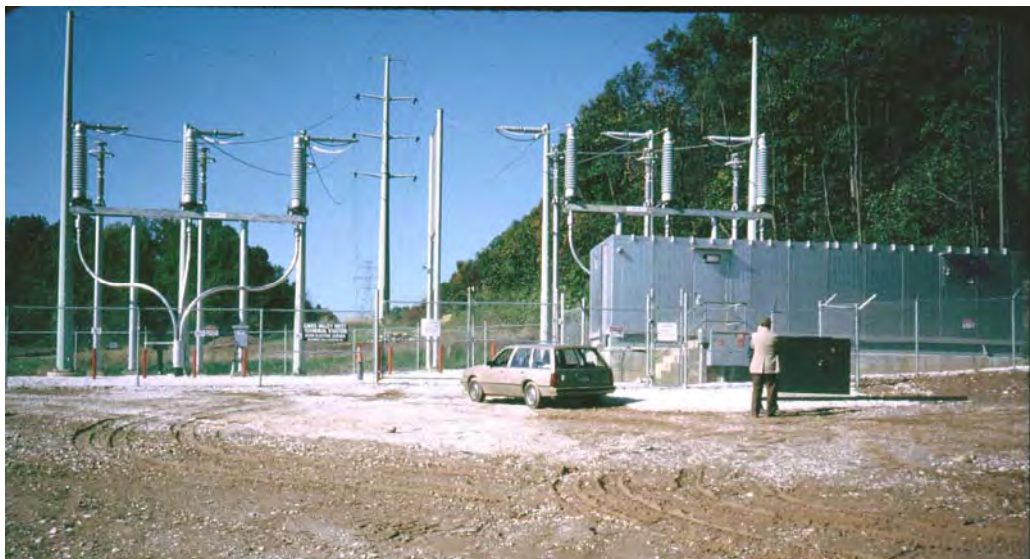
Figure 15. Typical 230 HPFF cable system transition station
