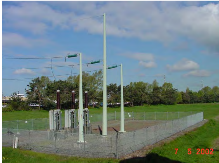
Figure 16. 230 kV SCFF overhead to underground transition with SCFF cables
