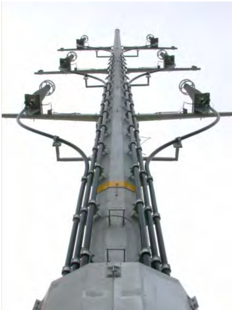
Figure 23. 230 kV overhead to underground transition using one steel riser pole for each of two circuits.
