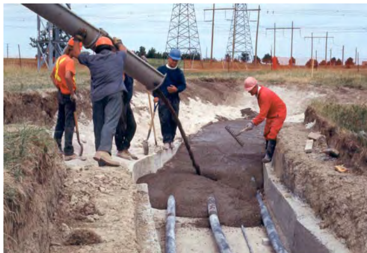
Figure 25. 230 kV XLPE transmission cable system construction
