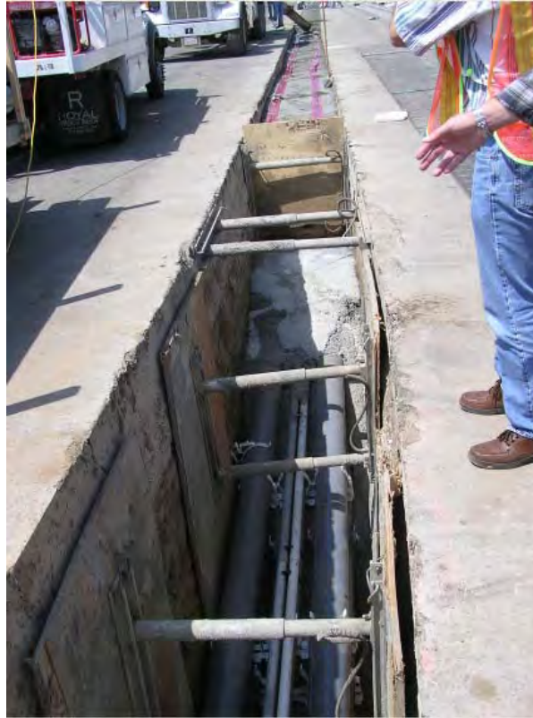
Figure 21. 230 kV XLPE transmission cable duct bank construction
