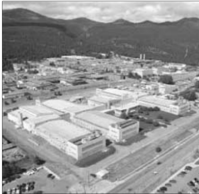
Figure 1B1 CMR Building
