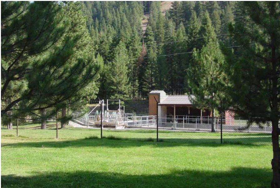
19. View from Imnaha River Road looking east* * Simulation view
