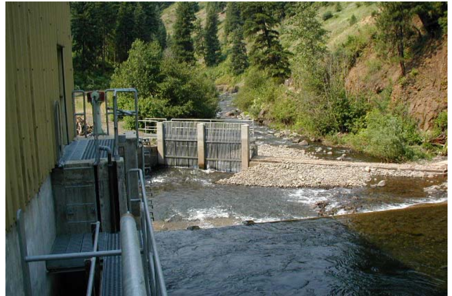
2. View of Lookingglass intake/downstream (not part of this project)
