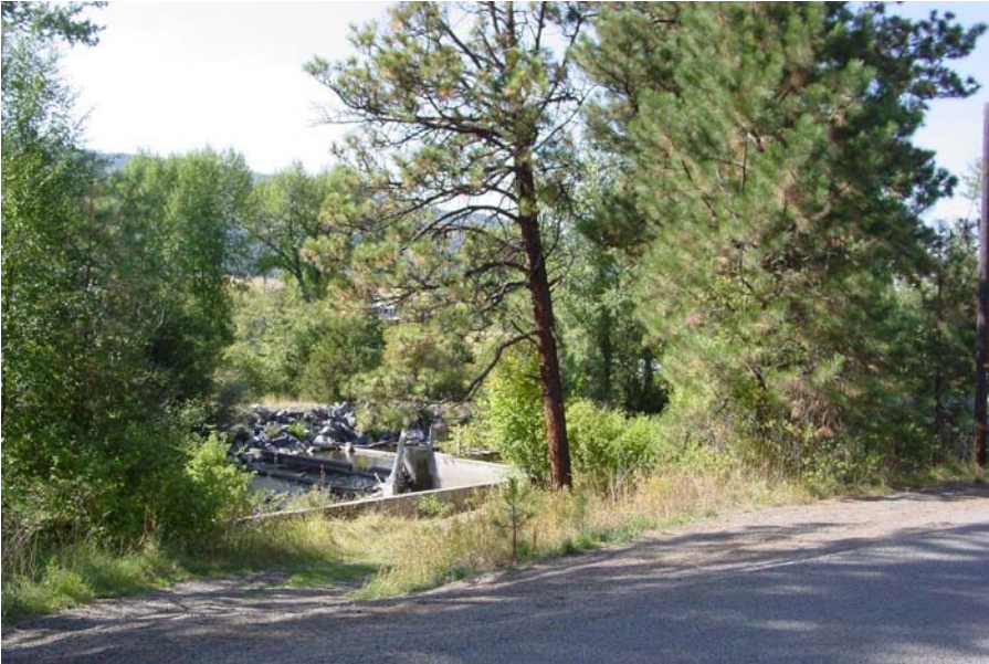
8. View from Lostine River Road (County Road 551) looking northwest*
