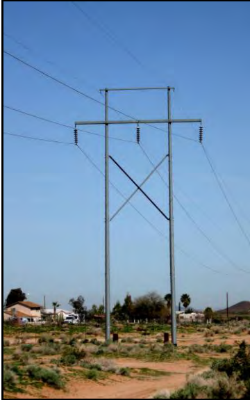
Photograph 2-1 Example of a Metal H-frame Structure
