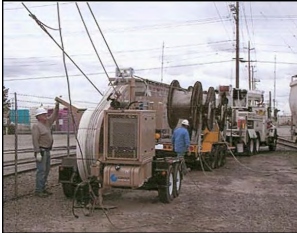
Photograph 2-9 Example of a Pulling Station
