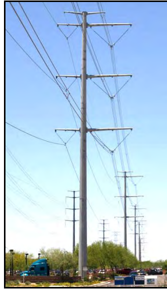
Photograph 2-4 Example of 500–230-kV Structure
