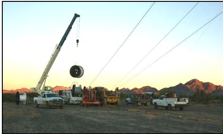
Photograph 2-5 Example of Tensioning Equipment
