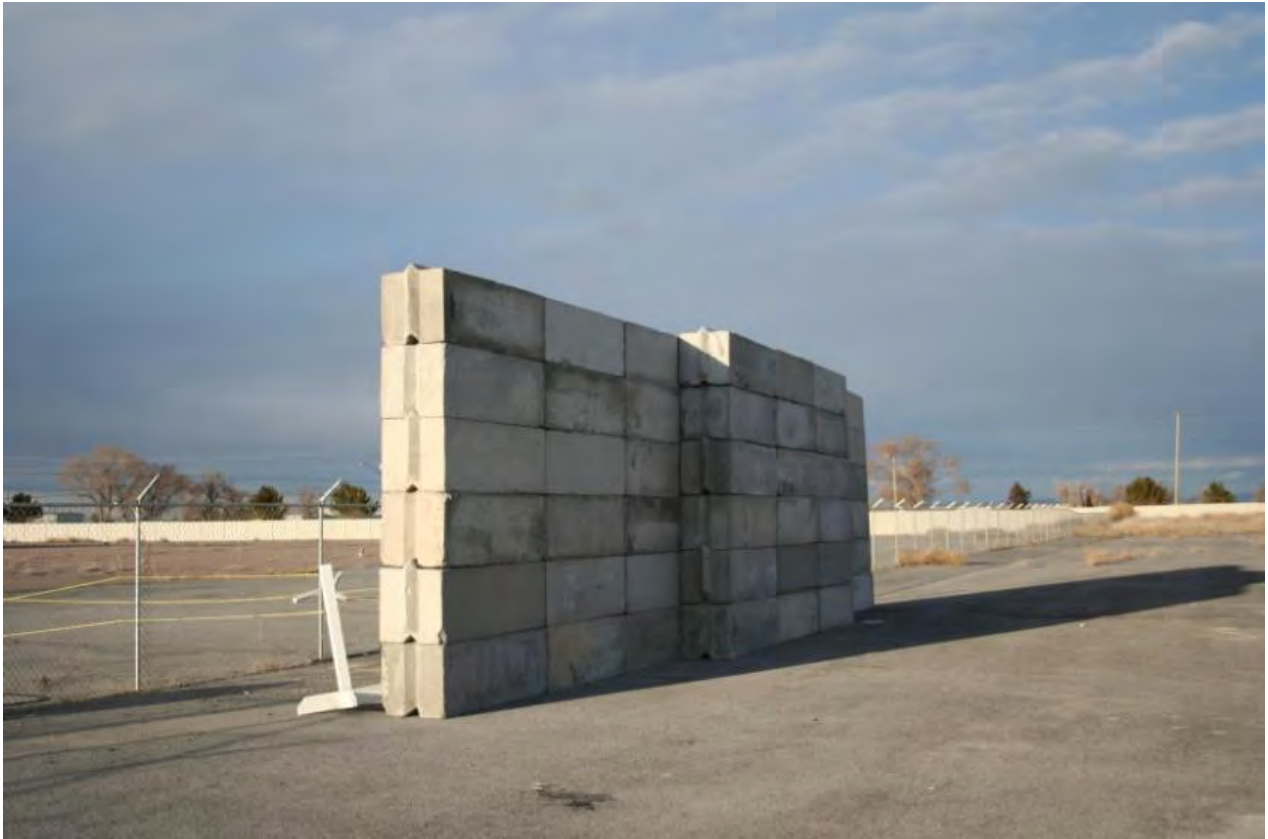
Figure A-5. Example of beam stop assembled using concrete blocks; this picture shows a typical beam stop for the Varitron-III shielding. Each block is 2 ft. thick, 2 ft. tall and 6 ft. long. The delivery and assembly of shield blocks requires semi trucks and forklifts; the movement of a large number of blocks usually only happens once every few years. For example, shield blocks could be placed in front of a trailer or control station pad, along the sides of the linac support building for uncollimated operations or so work could be conducted within the building, to prevent the beam from traveling outside the linac support building fenced area (see Figure A-3), or placed along the down range road to stop the beam from leaving the fenced portion of the SOX Range. This allows work with shorter beam lines, reducing the size of the radiologically control footprint or area.
