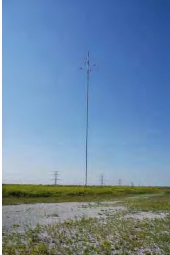
Photo 1: Existing meteorological tower on top of the demolition landfill (project site).
