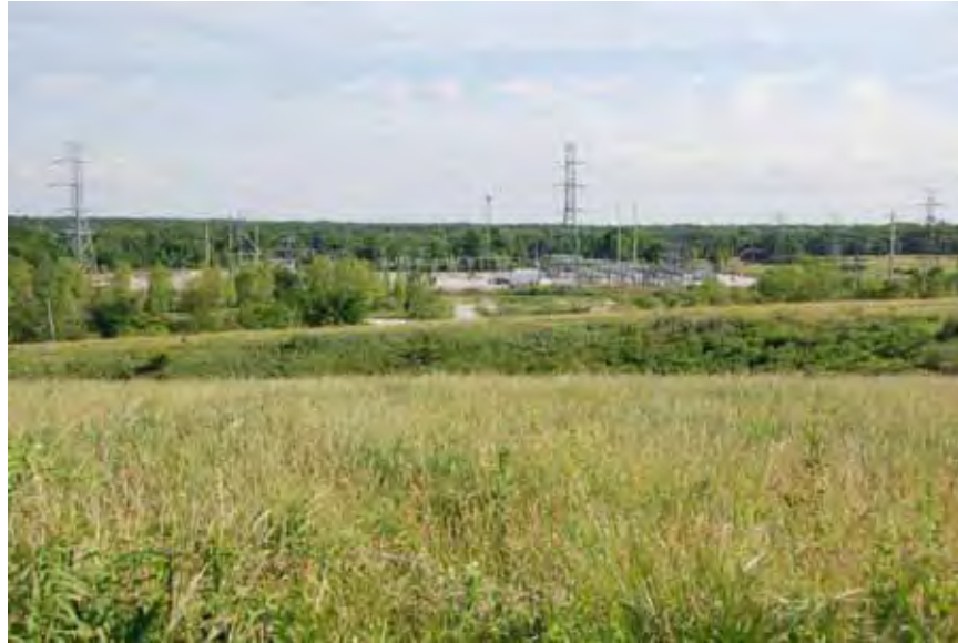
Photo 11: An electric substation south of the project area.
