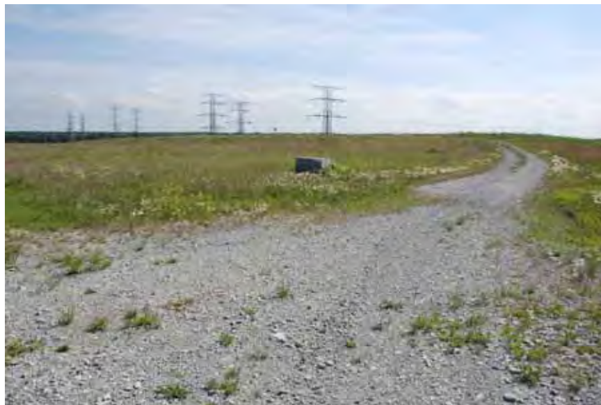
Photo 2: Access road to the top of the landfill.
