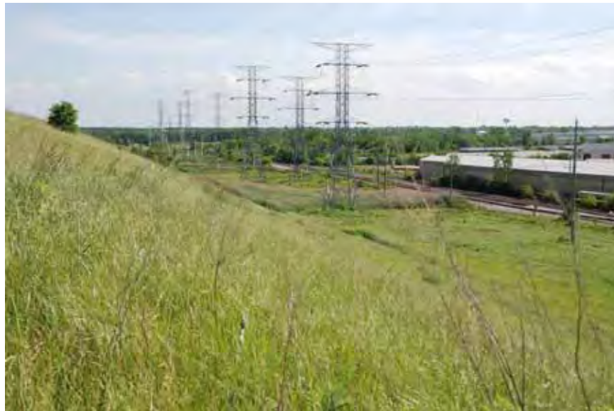
Photo 4: High voltage transmission lines and towers along the western boundary of the project site.
