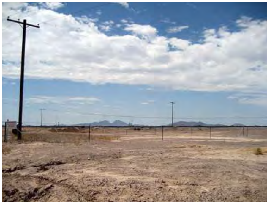
View looking north towards Mesquite Generating Station and gen-tie route.
