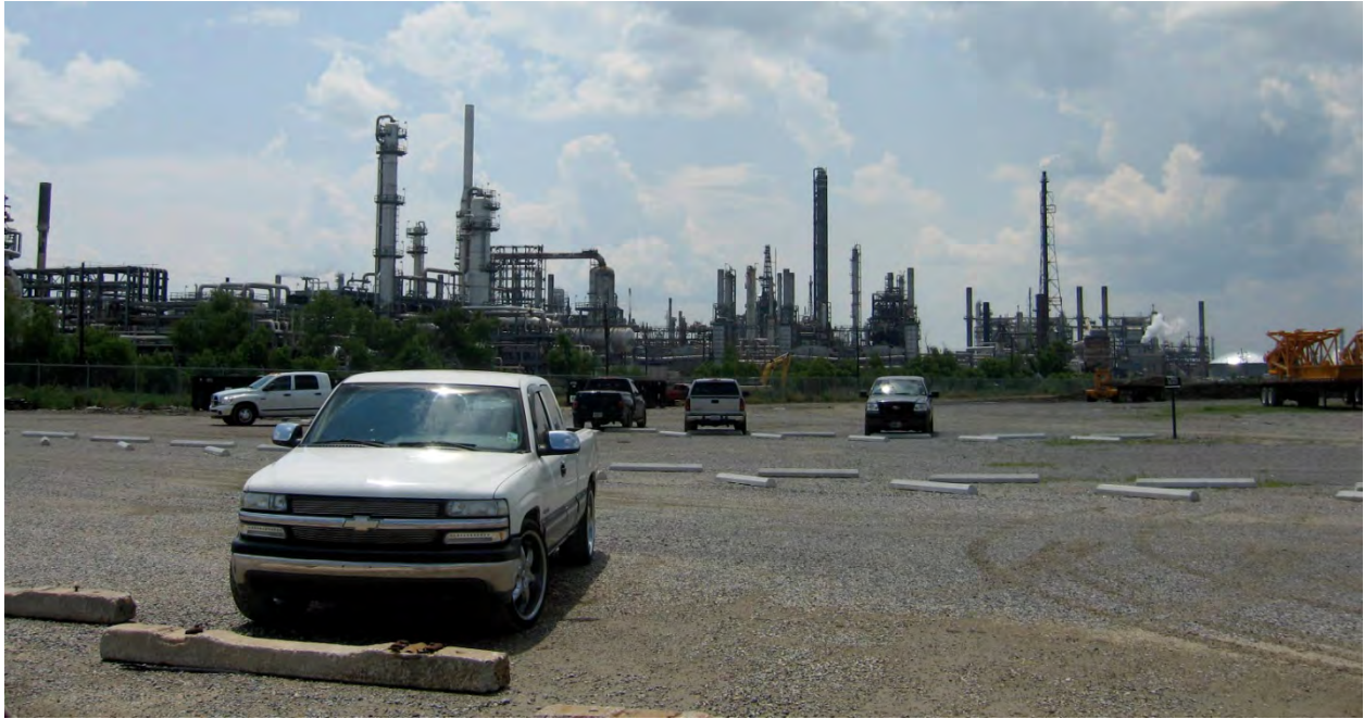
Picture 1: Twenty acre plant site (looking across site towards Valero St. Charles Refinery).
