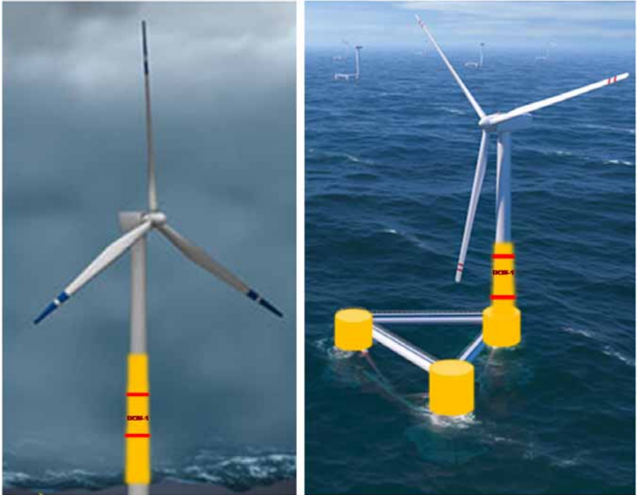
Figure 3-19. Proposed Paint Scheme and Marking of Spar Buoy (or TLP) Platform (left) and Semi-Submersible Platform (right)
