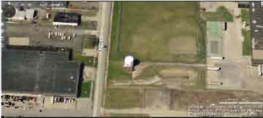
35'-high EP3 water tower on Lincoln Electric Company property, 562' (0.106 mi) SSW of proposed wind turbine
