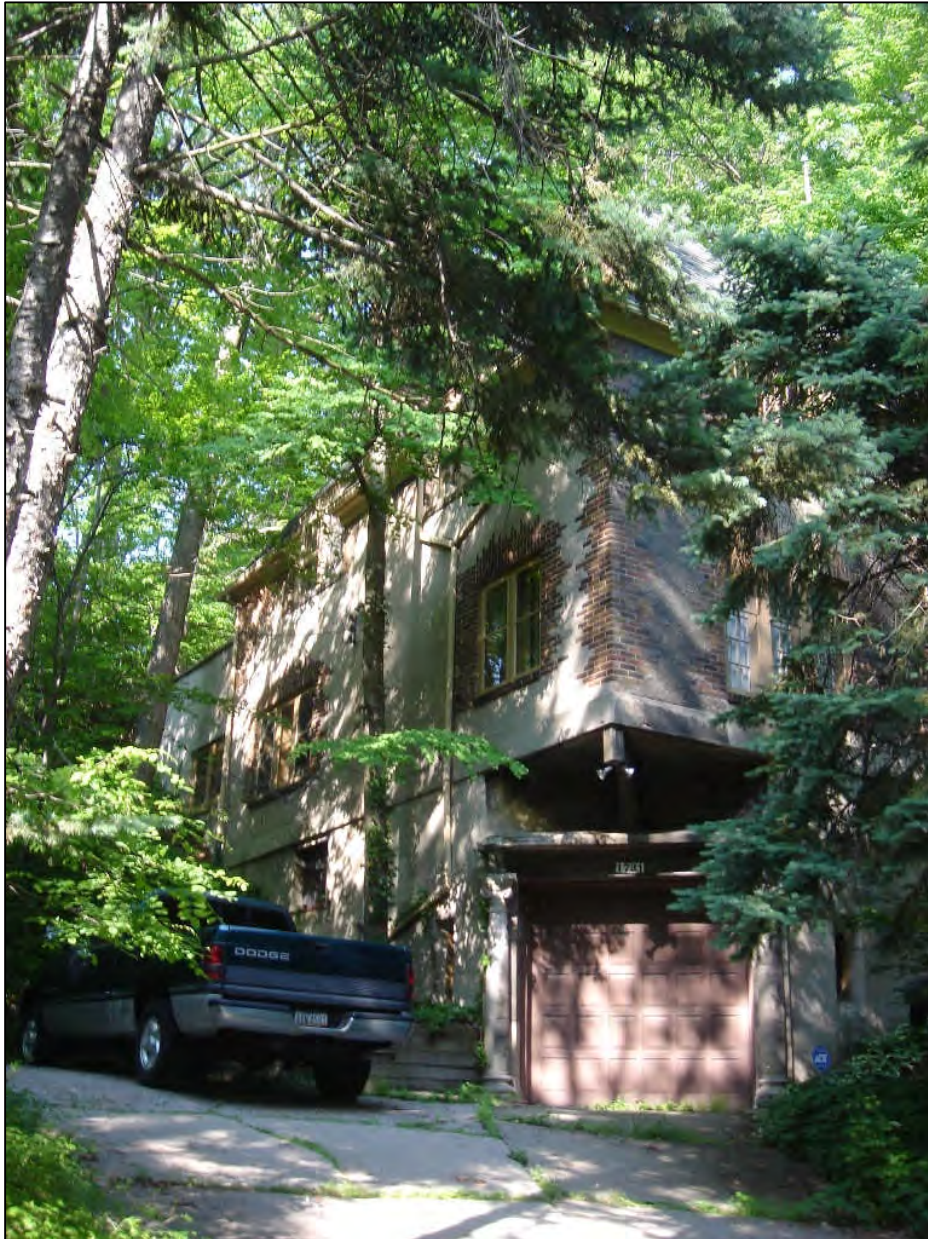
1731 Beverly Hills Drive, CUY-01651-22, Southwest Elevation
