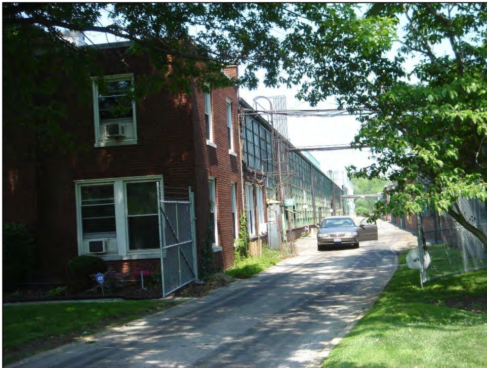
Ajax Manufacturing Co., CUY-01652-22, West Elevation
