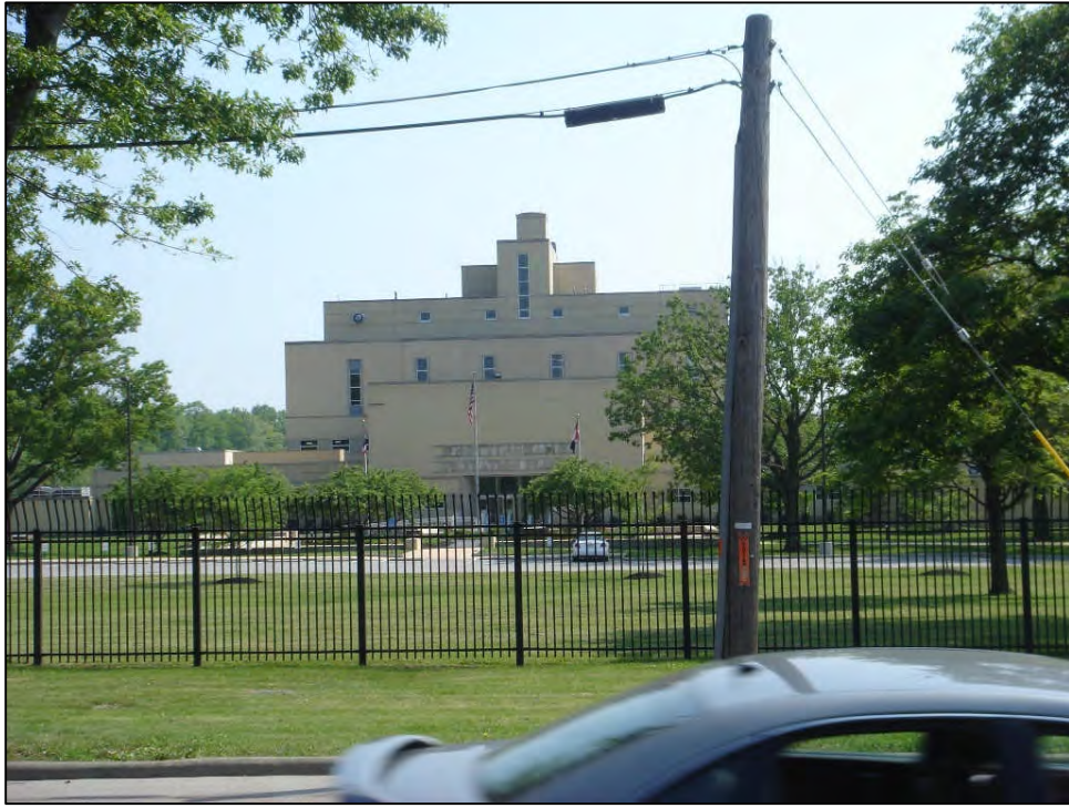
Nottingham Filtration Plant, CUY-01659-22, South Elevation
