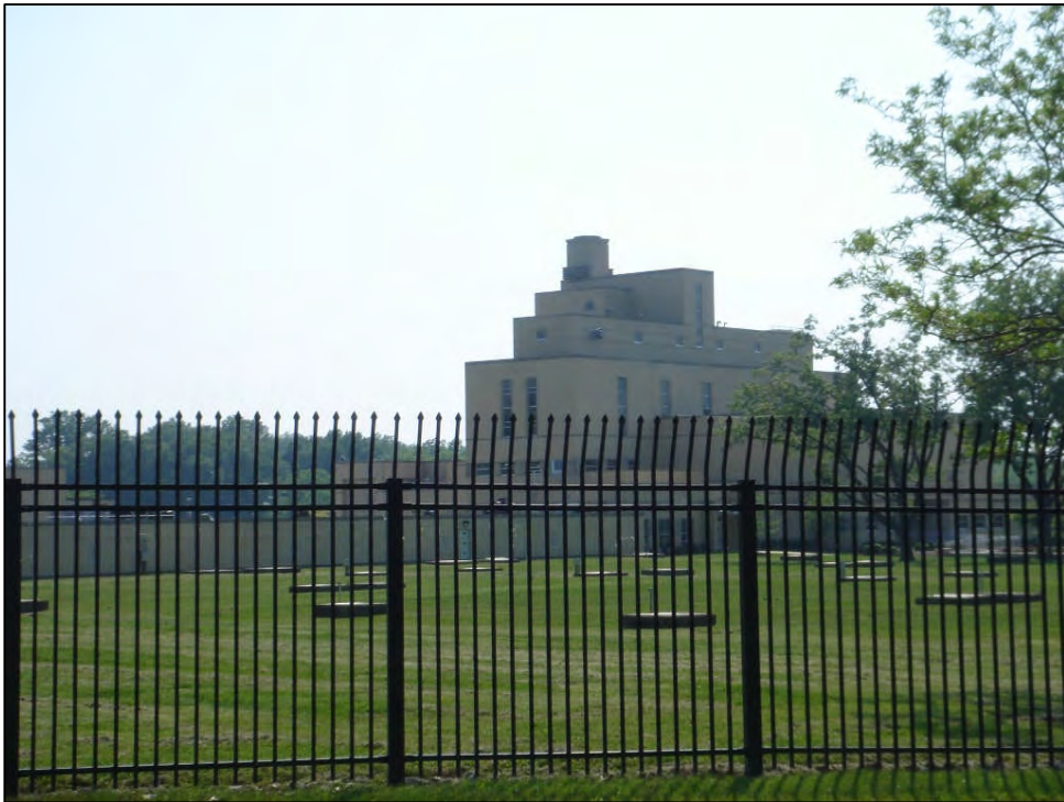
Nottingham Filtration Plant, CUY-01659-22, Southeast Elevation
