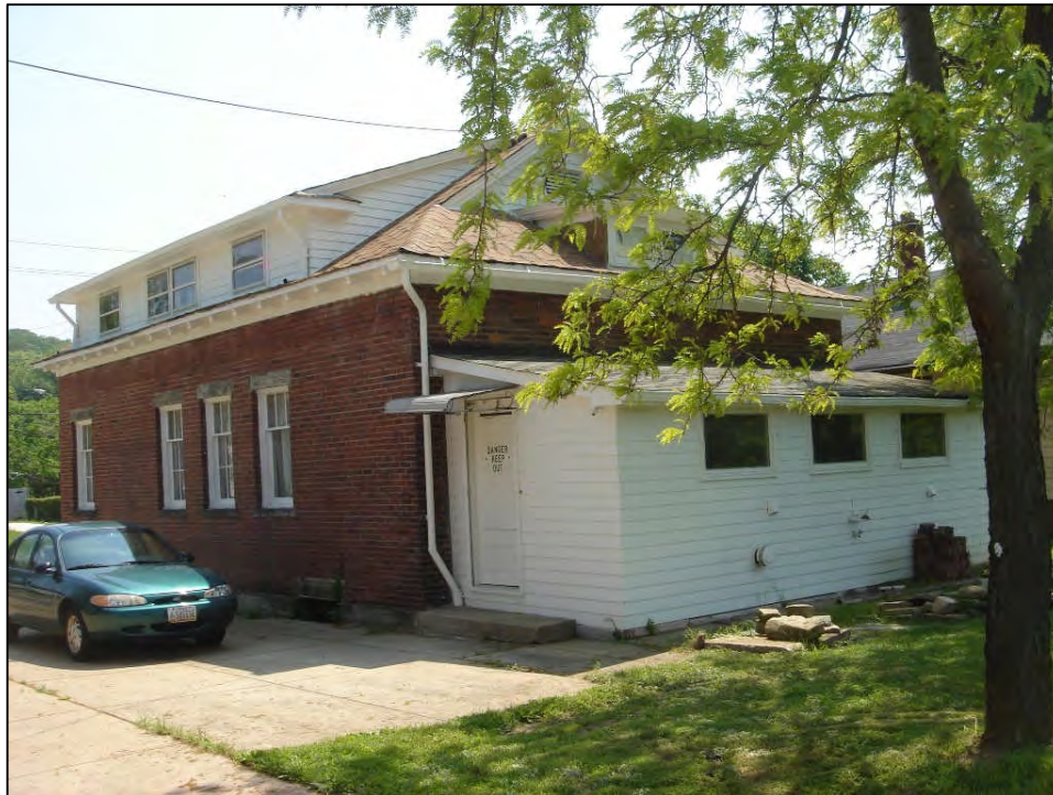
North Street School, CUY-01652-22, Northeast Elevation
