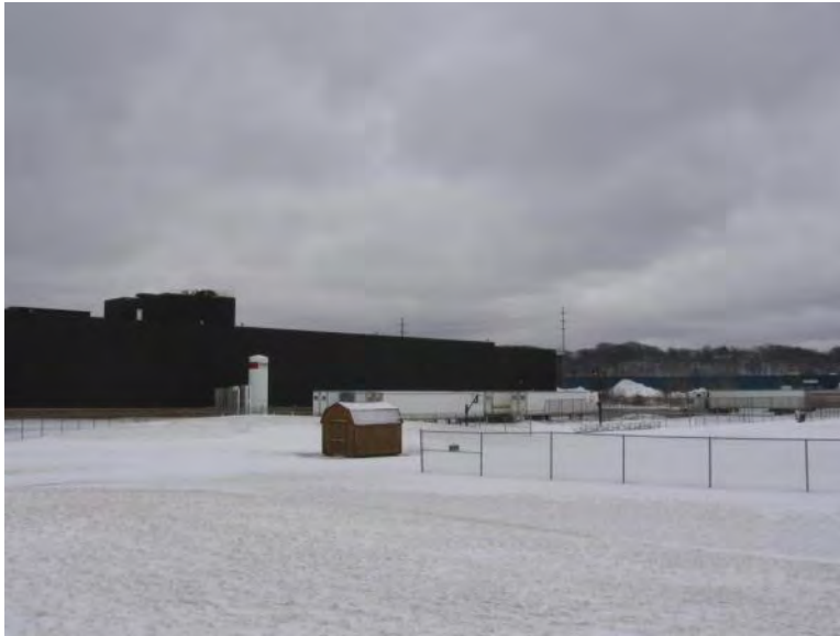
Figure 6: Turbine location looking southeast at Lincoln-owned building. Note absence of windows.
