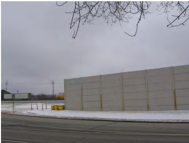
Figure 13: Photo Location 1 looking toward turbine, highway noise barrier ~20+ feet tall
