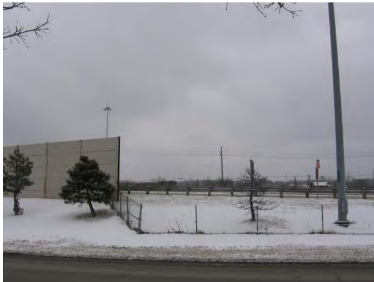
Figure 15: Photo Location 1 looking toward turbine, noise barrier ~20+ feet tall
