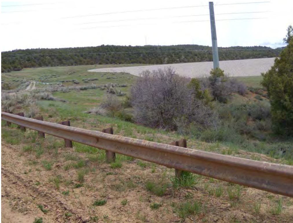
Figure 6. View of the Durango Disposal Site Looking North from CR 212 (Transmission lines and a pole are visible in the foreground.)
