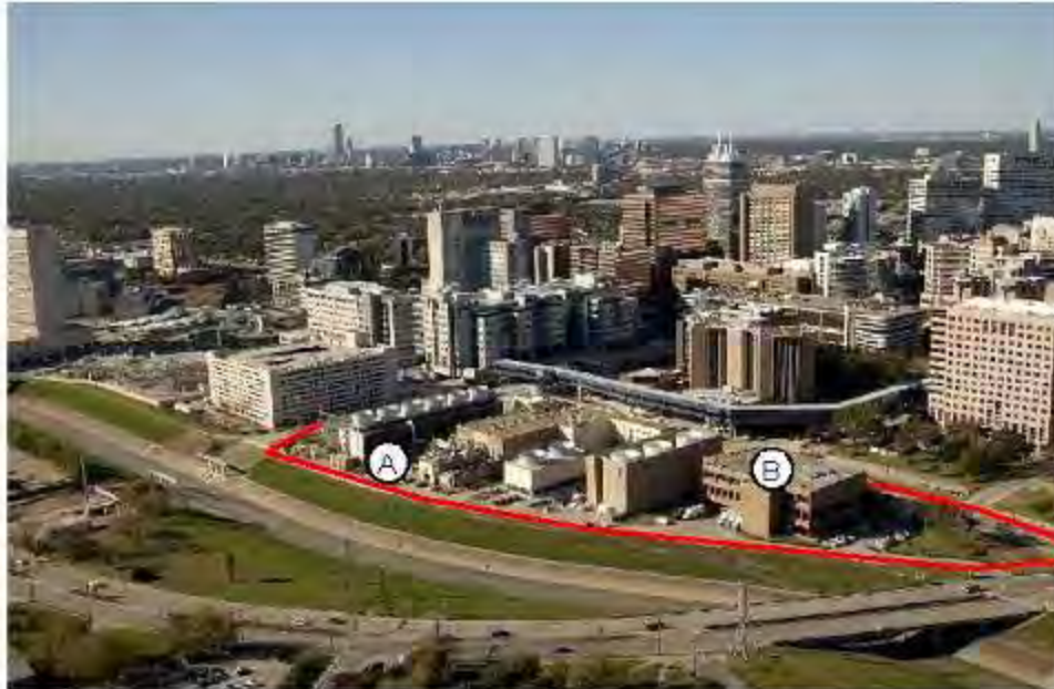
Figure 3. Thermal Energy Corporation Central Plant (outlined in red) (view to northwest). The CHP gas turbine and heat recovery steam generator will be installed near the southern boundary of the property (A). The chillers will be installed in a building currently being constructed on eastern portion of the property (B), where the recently removed Texas Medical Center laundry is shown in this photograph.
