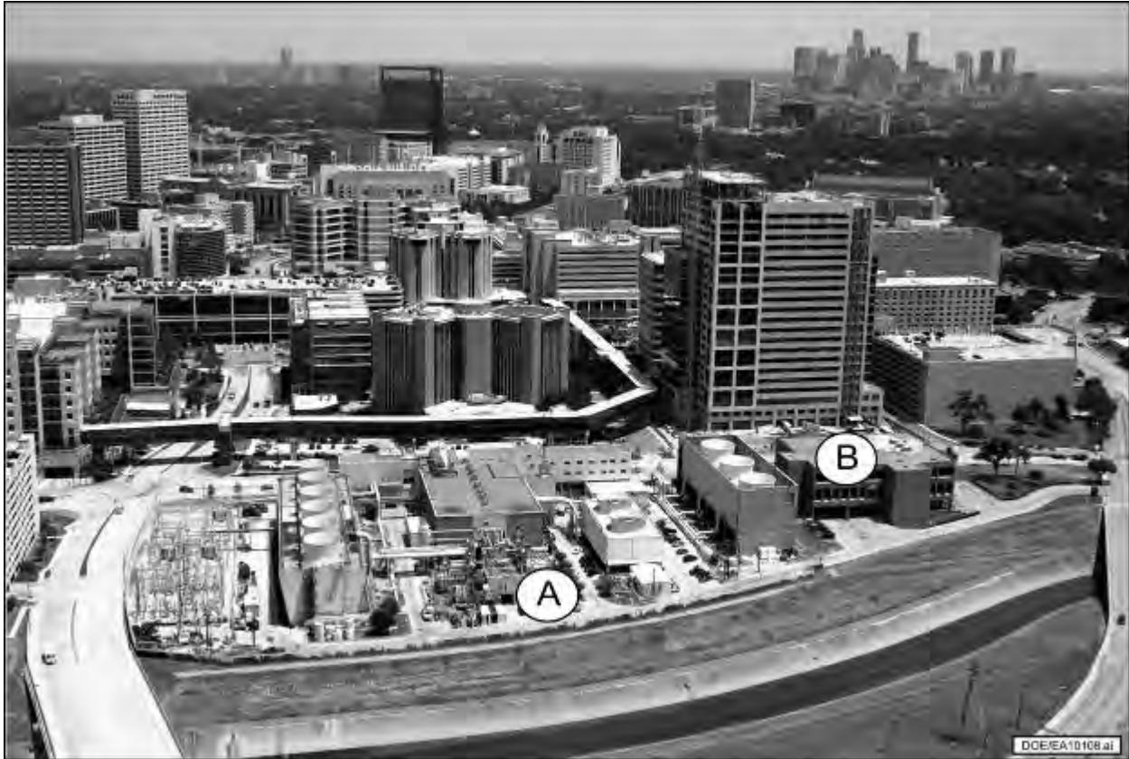
Figure 2-2. The TECO Central Plant prior to expansion and upgrades (view to north). TECO would install the CHP system near the southern boundary of the facility (A) and the four new water chillers in a building being constructed where the laundry facility (B) is shown in this photograph.
