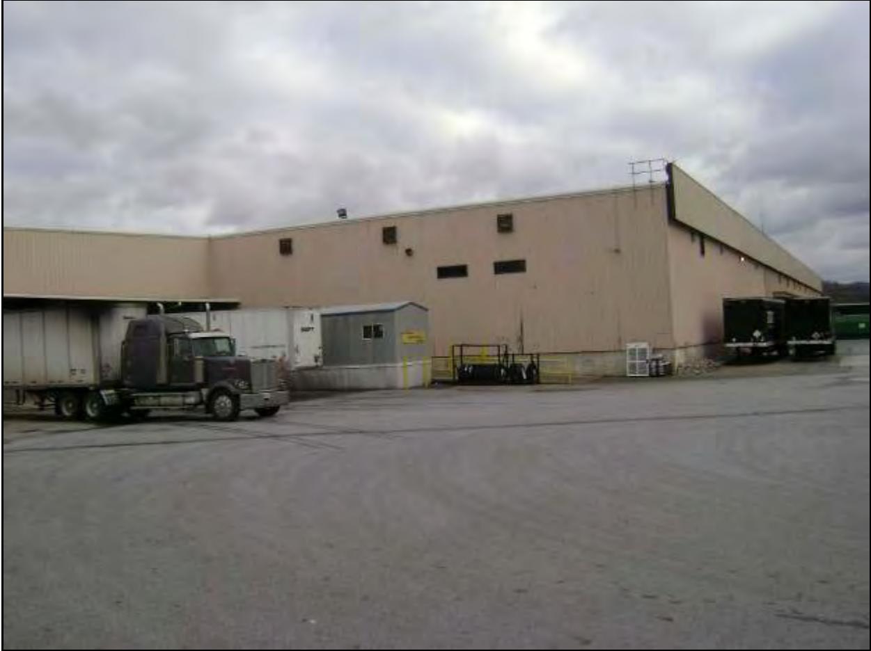
Figure 2-4. View of the south and west sides of the Bristol plant building. Exide would modify a portion of the building (to the rear in this view) for the proposed operations.
