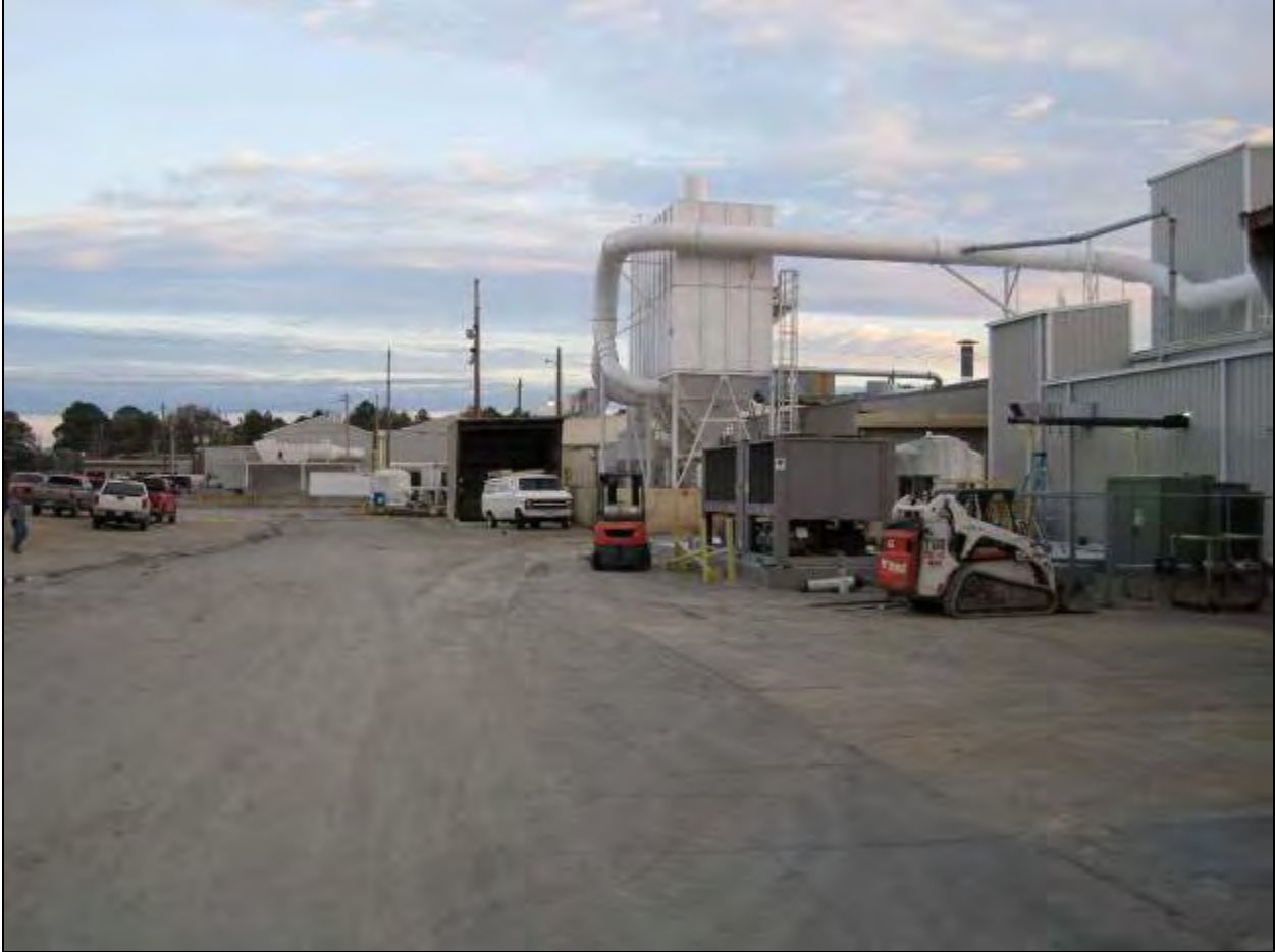
Figure 2-6. View of the south side of the proposed Columbus project area. Exide would remove the baghouse, demolish the building to the right, and then construct the addition in this area.
