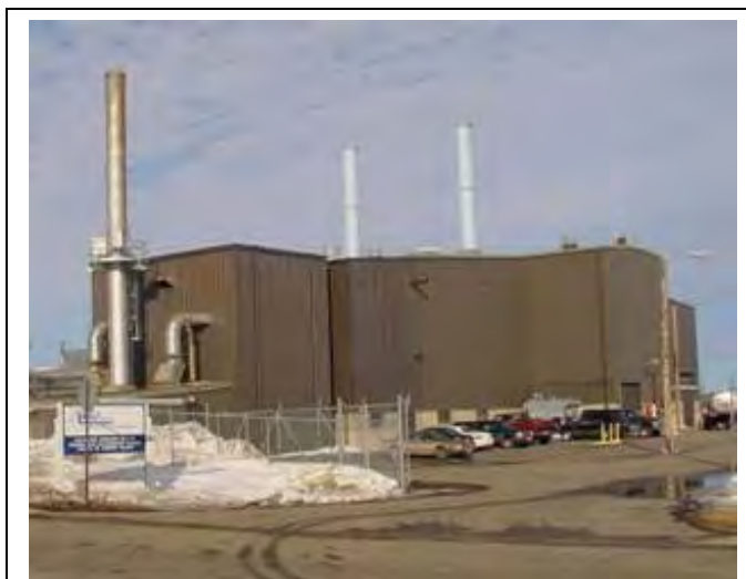
Figure 1-1. PDSWM Waste-to-Energy Facility
