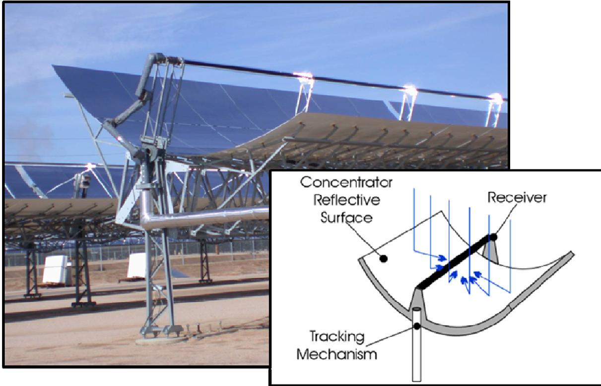
Figure 2-2 Parabolic Trough<sup>3</sup>
