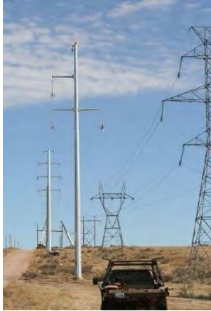
Typical-style monopole structure and monopole with “weathering” steel finish.
