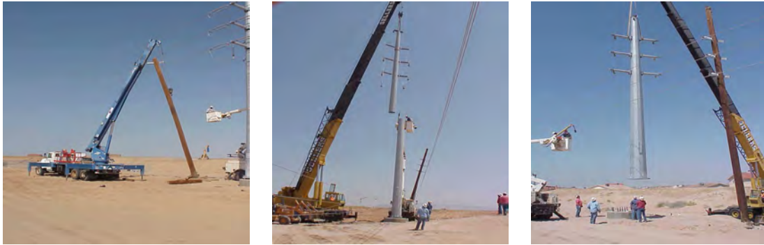
Typical monopole structure placement, with crews and equipment at work at the structure site.
