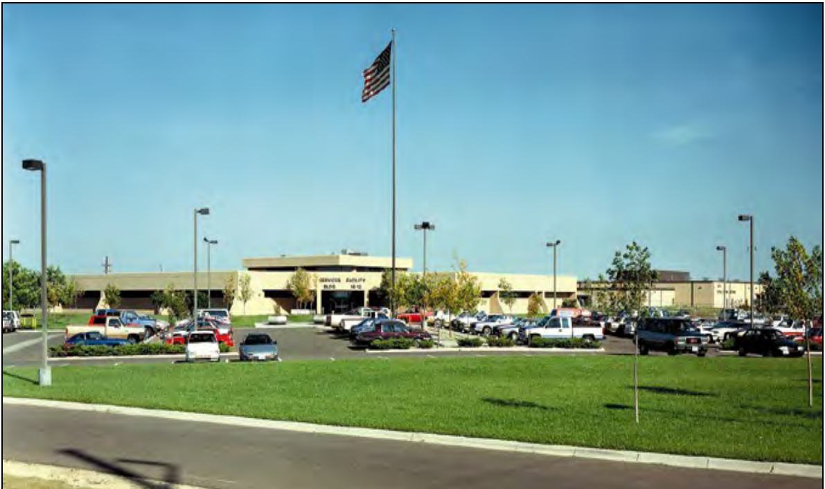
PANTEX PLANT * AMARILLO, TEXAS * JUNE 2008
