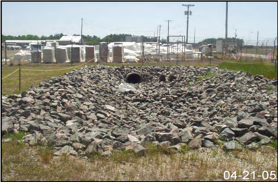
Figure 2-78. View of Stormwater Outfall N-2A.
