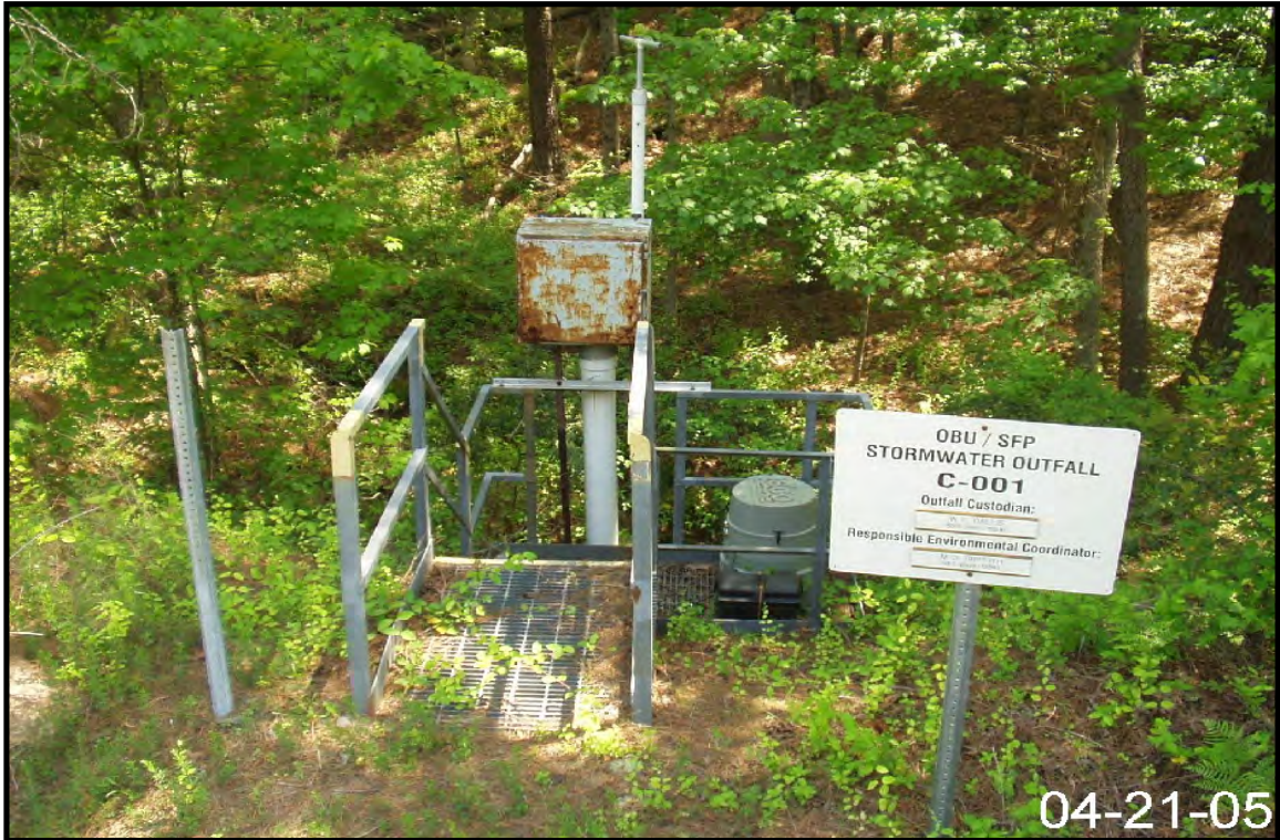
Figure 2-9. View of Stormwater Outfall C-01.
