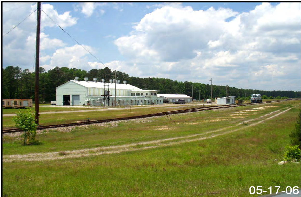
Figure 2-121. Representative View of Drainage Area for Stormwater Outfall Y-01.
