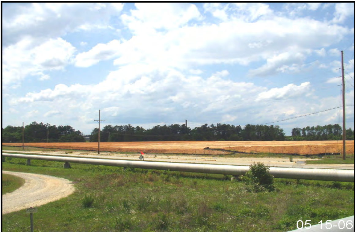
Figure 2-28. Representative View of Drainage Area for Stormwater Outfall E-05.
