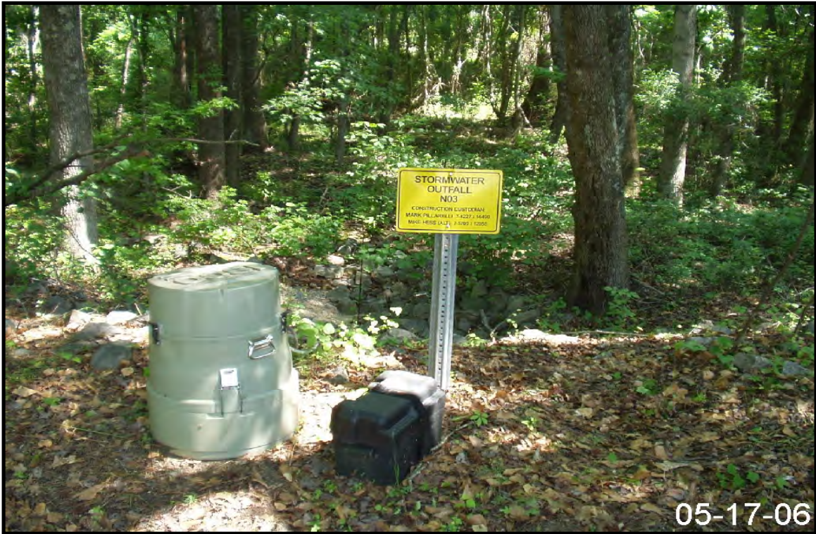
Figure 2-81. View of Stormwater Outfall N-03.
