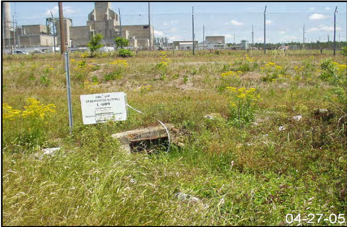
Figure 2-65. View of Stormwater Outfall L-09.
