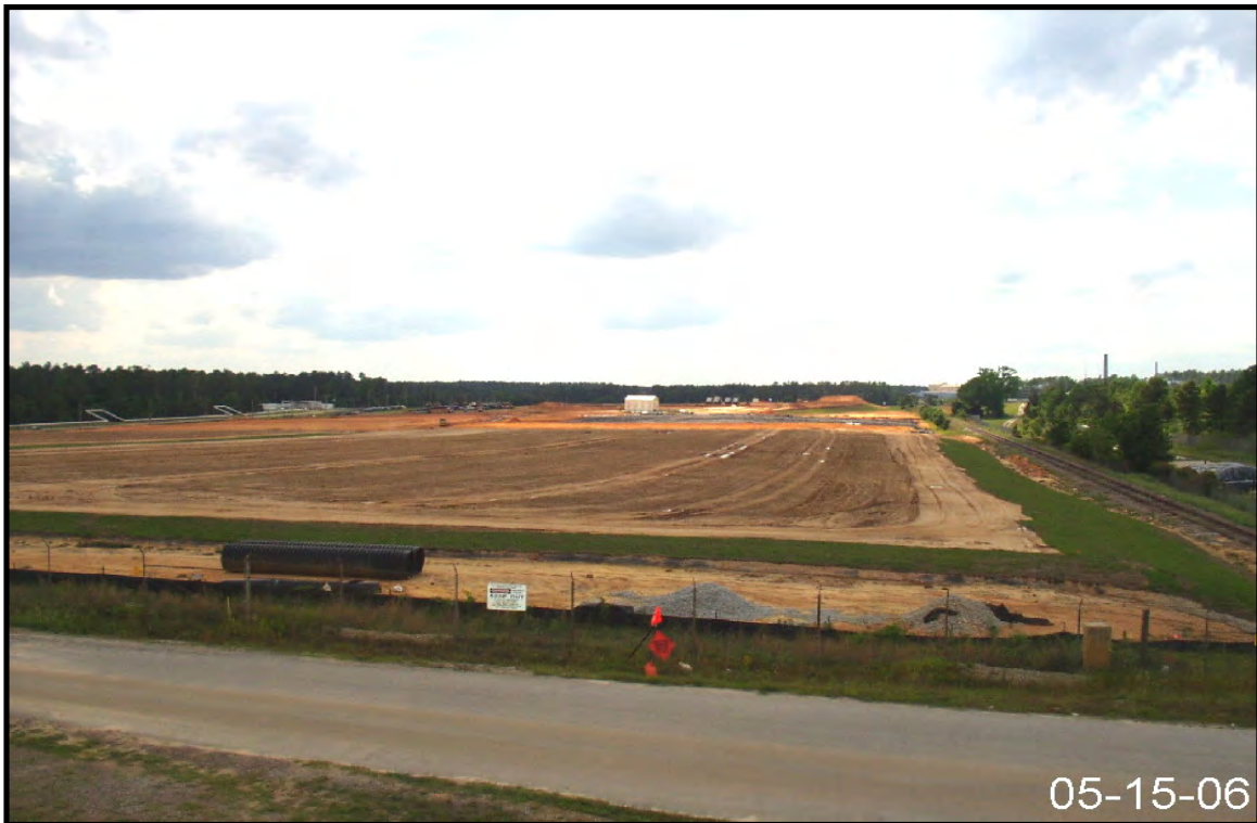
Figure 2-16. Representative View of Drainage Area for Stormwater Outfall E-01.
