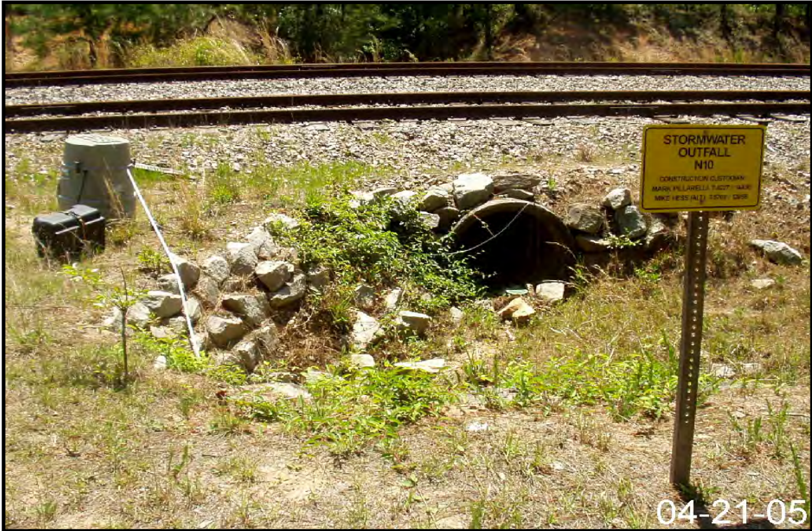
Figure 2-90. View of Stormwater Outfall N-10.
