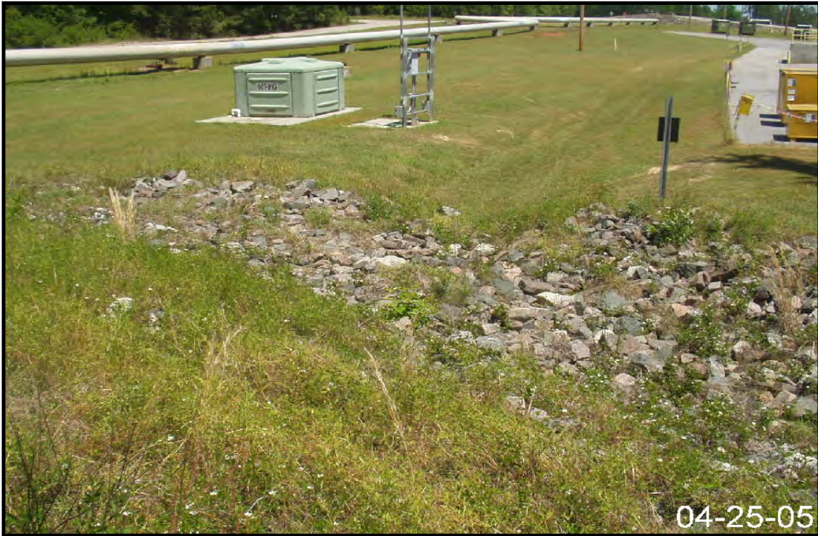
Figure 2-36. View of Stormwater Outfall FT-01.
