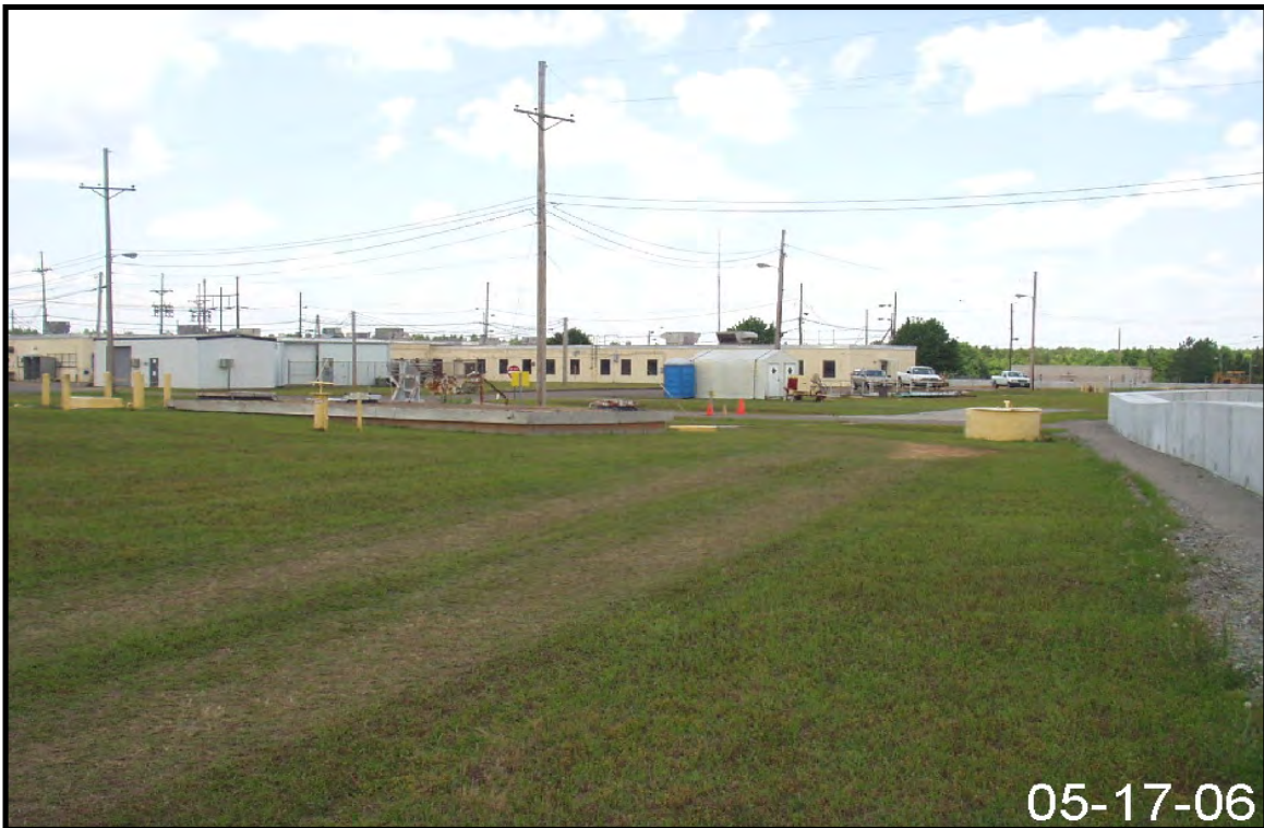
Figure 2-56. Representative View of Drainage Area for Stormwater Outfall K-02.
