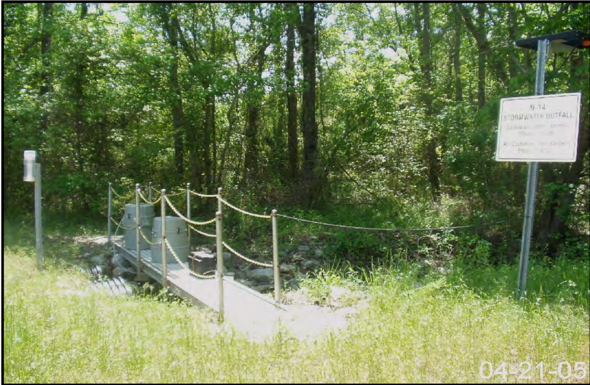
Figure 2-102. View of Stormwater Outfall N-14.
