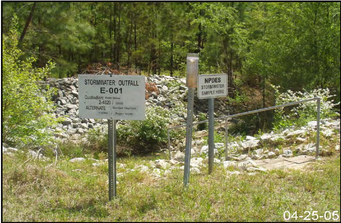
Figure 2-15. View of Stormwater Outfall E-01.
