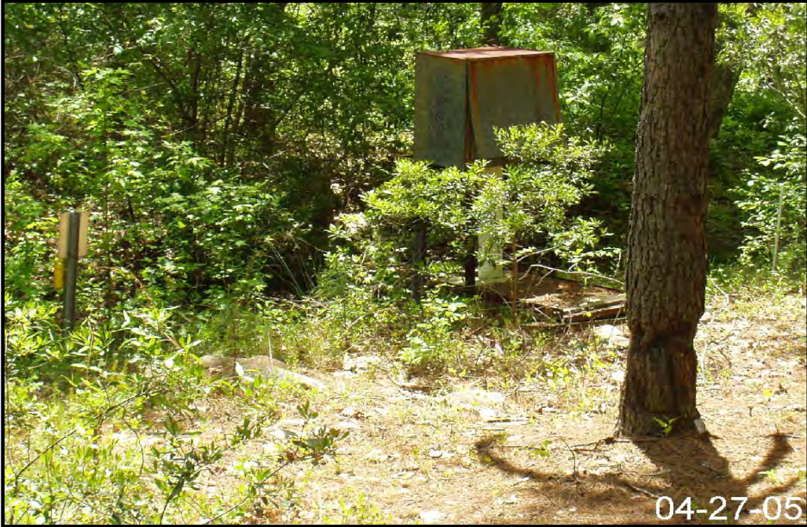
Figure 2-114. View of Stormwater Outfall P-13.
