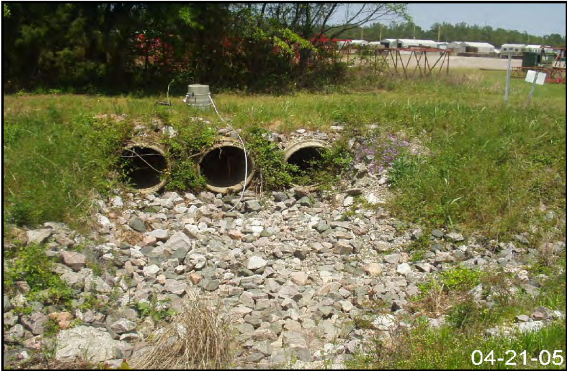
Figure 2-93. View of Stormwater Outfall N-12.
