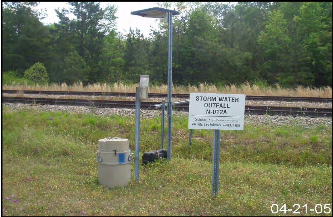
Figure 2-97. View of Stormwater Outfall N-12A.
