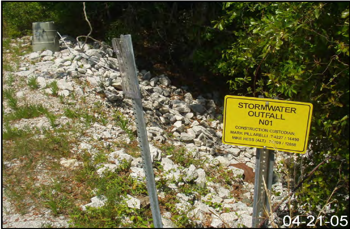
Figure 2-71. View of Stormwater Outfall N-01.
