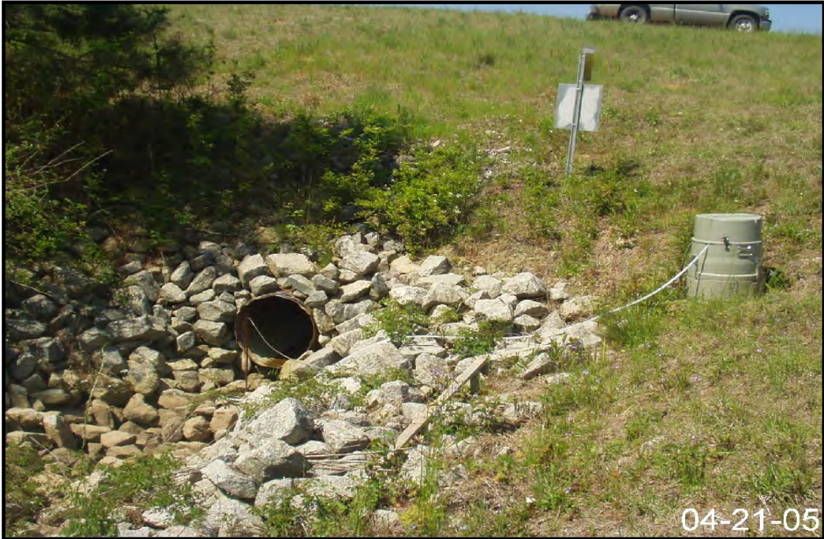
Figure 2-33. View of Stormwater Outfall F-3B.
