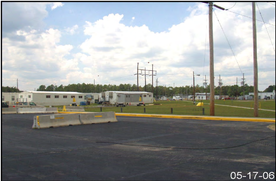
Figure 2-66. Representative View of Drainage Area for Stormwater Outfall L-09.
