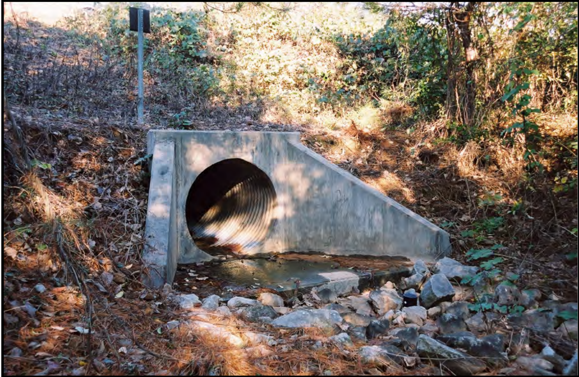
Figure 2-21. View of Stormwater Outfall E-03.
