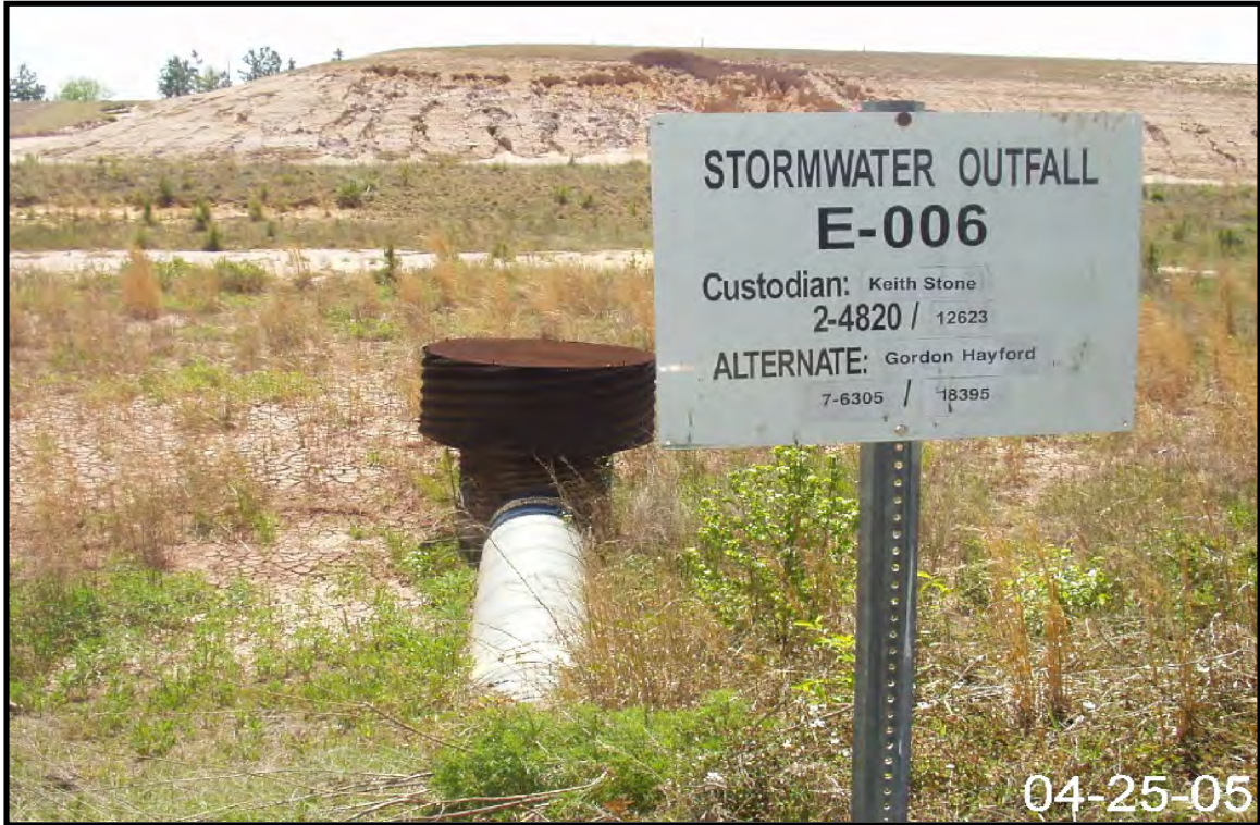
Figure 2-30. View of Stormwater Outfall E-06.
