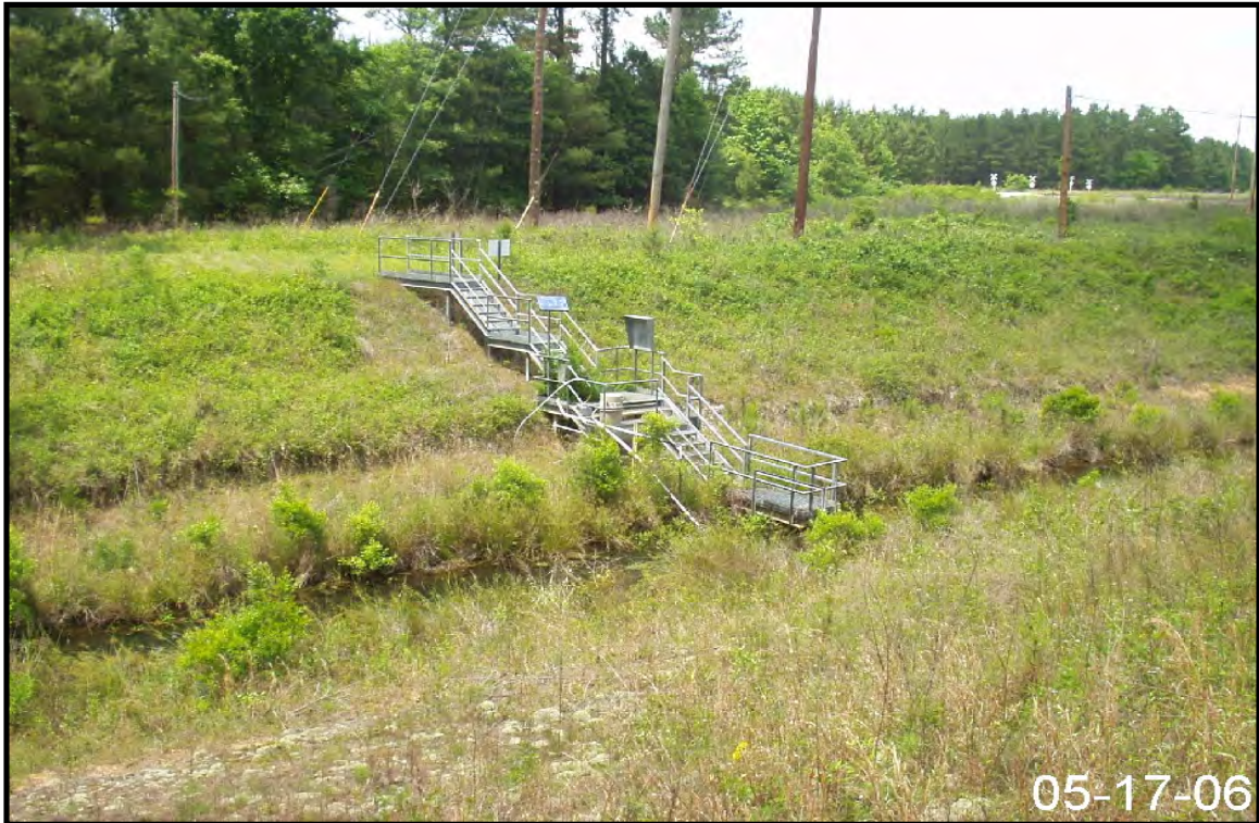
Figure 2-117. View of Stormwater Outfall P-19.
