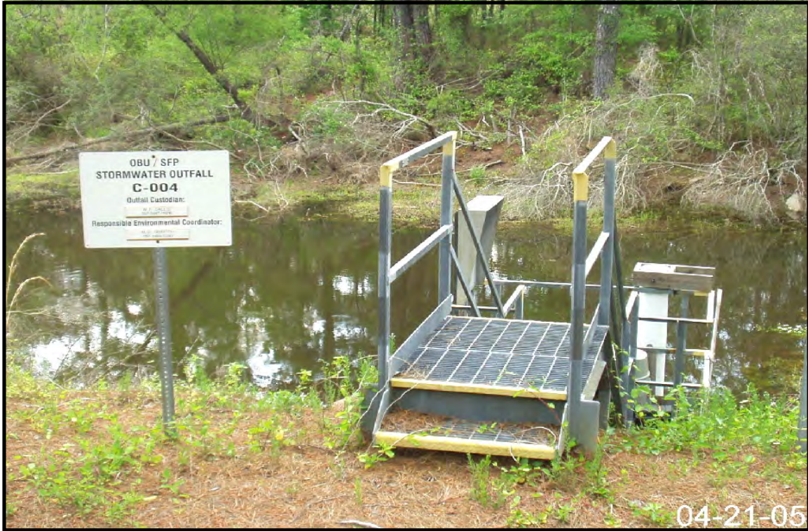
Figure 2-12. View of Stormwater Outfall C-04.
