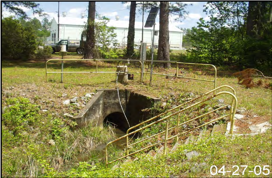
Figure 2-120. View of Stormwater Outfall Y-01.
