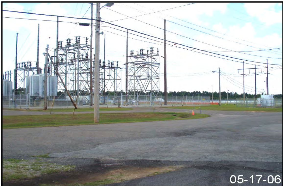
Figure 2-52. Representative View of Drainage Area for Stormwater Outfall K-01.
