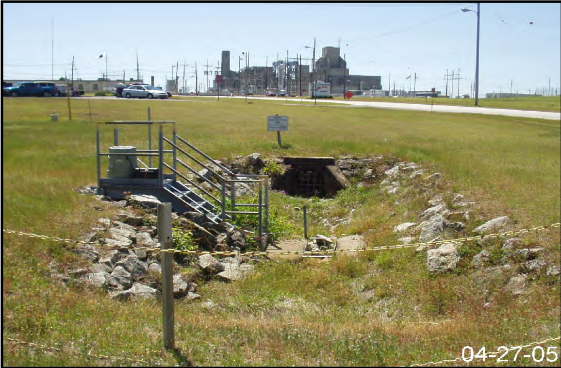
Figure 2-51. View of Stormwater Outfall K-01.
