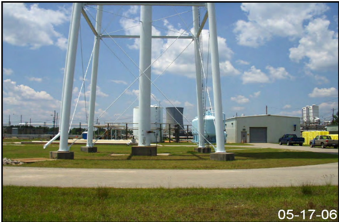
Figure 2-60. Representative View of Drainage Area for Stormwater Outfall K-04.
