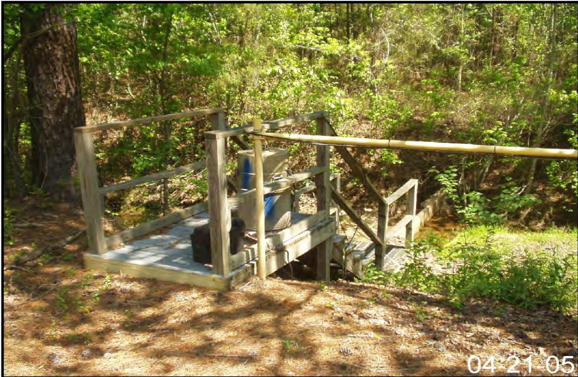
Figure 2-87. View of Stormwater Outfall N-06.
