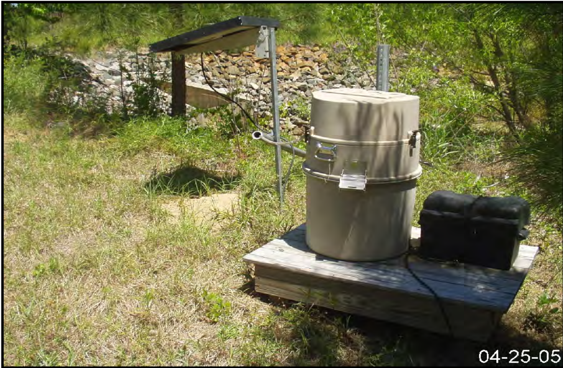
Figure 2-27. View of Stormwater Outfall E-05.
