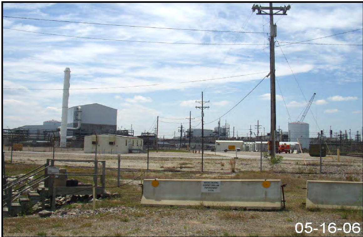
Figure 2-43. Representative View of Drainage Area for Stormwater Outfall H-7A.
