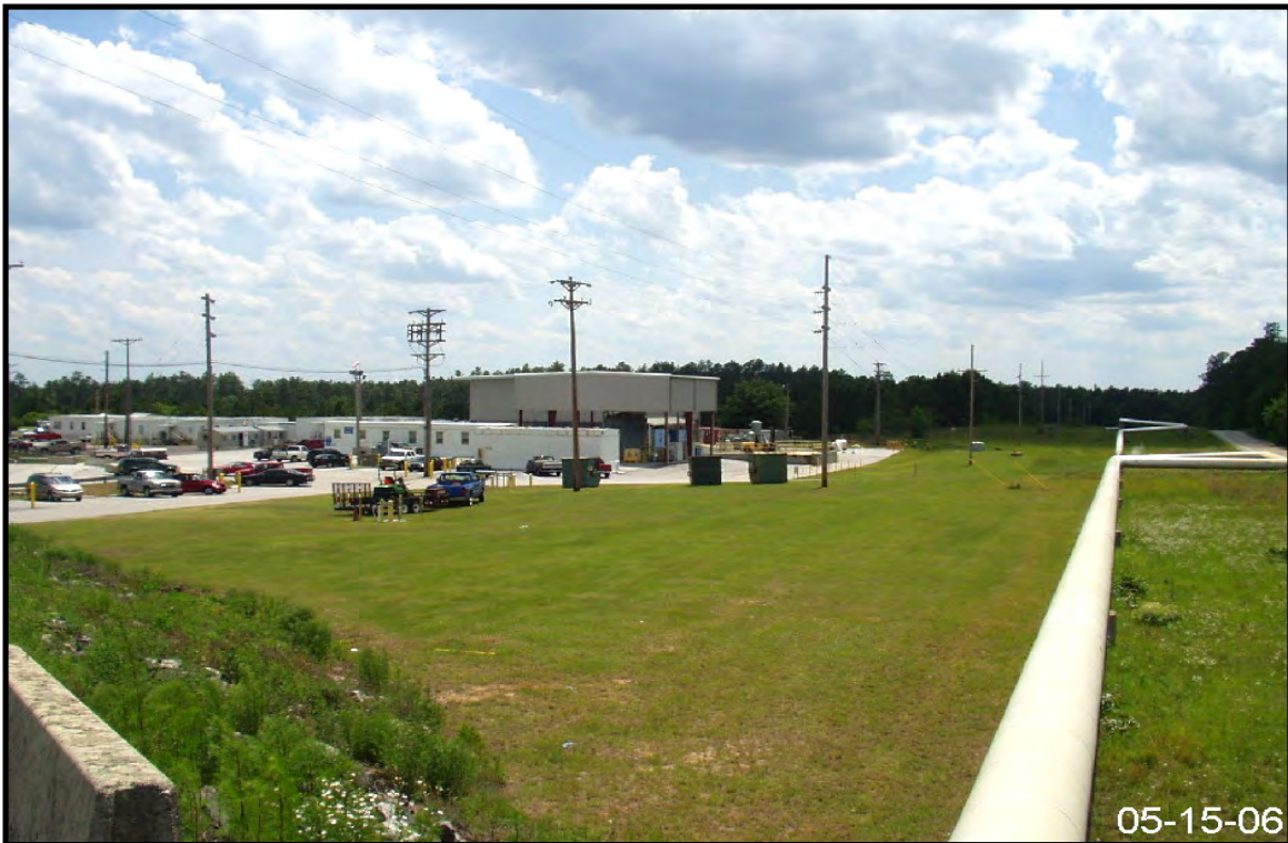
Figure 2-37. Representative View of Drainage Area for Stormwater Outfall FT-01.
