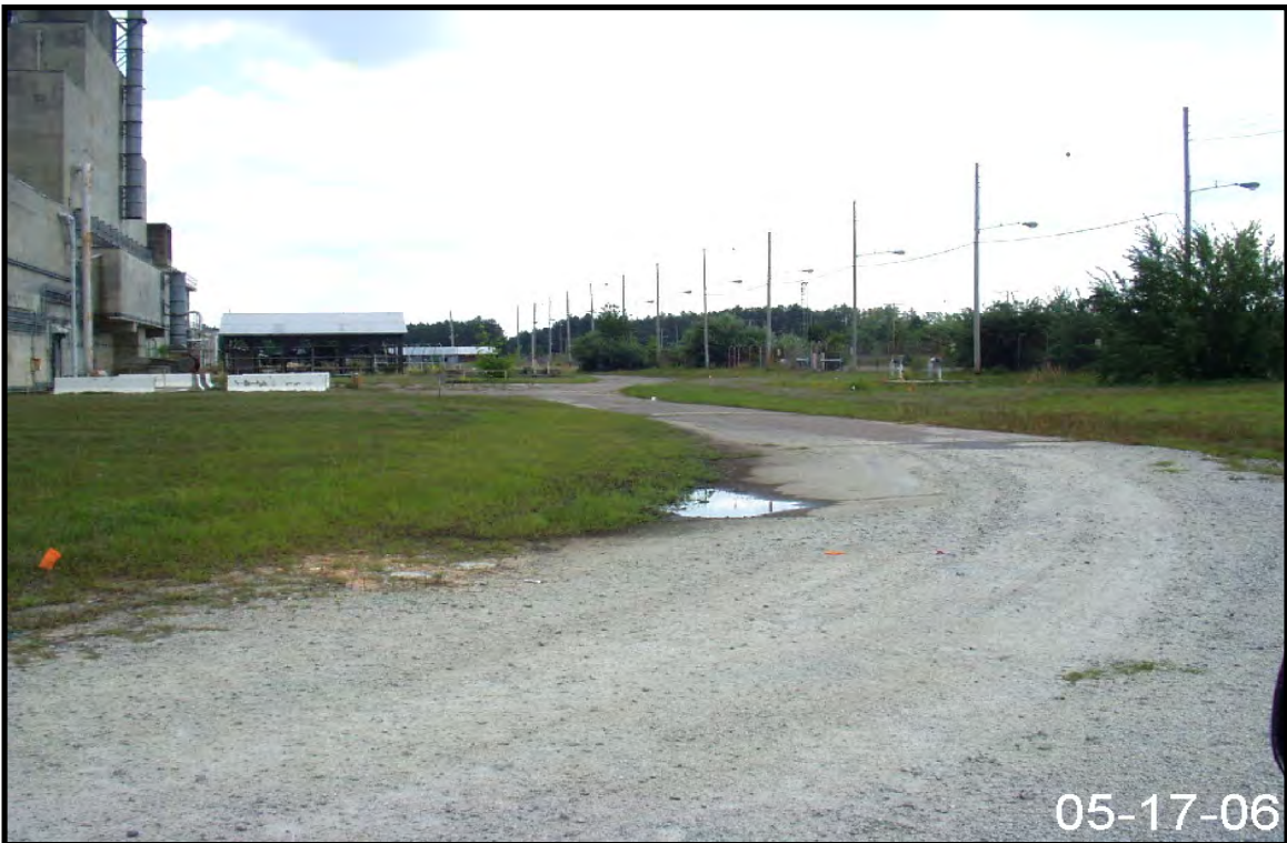
Figure 2-118. Representative View of Drainage Area for Stormwater Outfall P-19.
