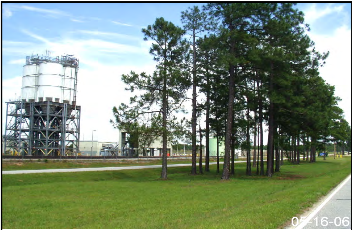
Figure 2-127. Representative View of Drainage Area for Stormwater Outfall Z-01.
