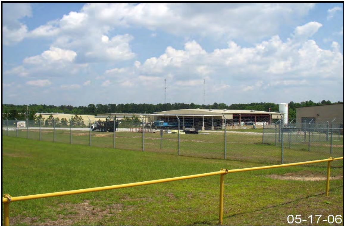
Figure 2-109. Representative View of Drainage Area for Stormwater Outfall N-16.
