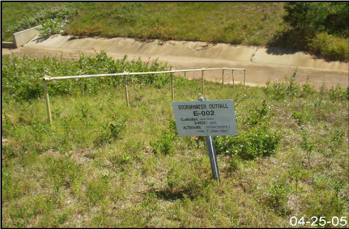
Figure 2-18. View of Stormwater Outfall E-02.
