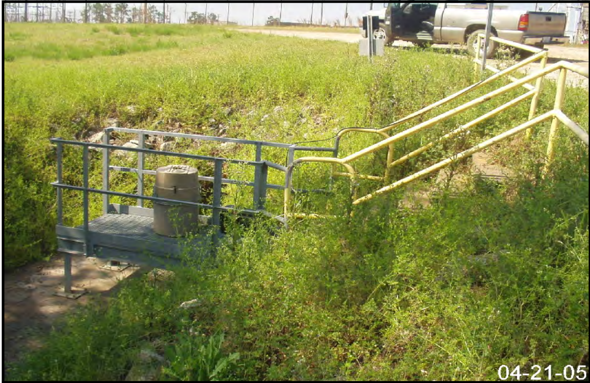
Figure 2-3. View of Stormwater Outfall A-08.
