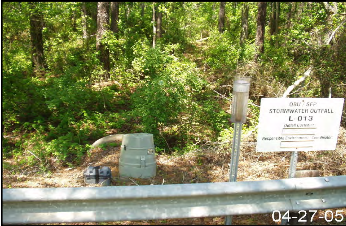
Figure 2-68. View of Stormwater Outfall L-13.
