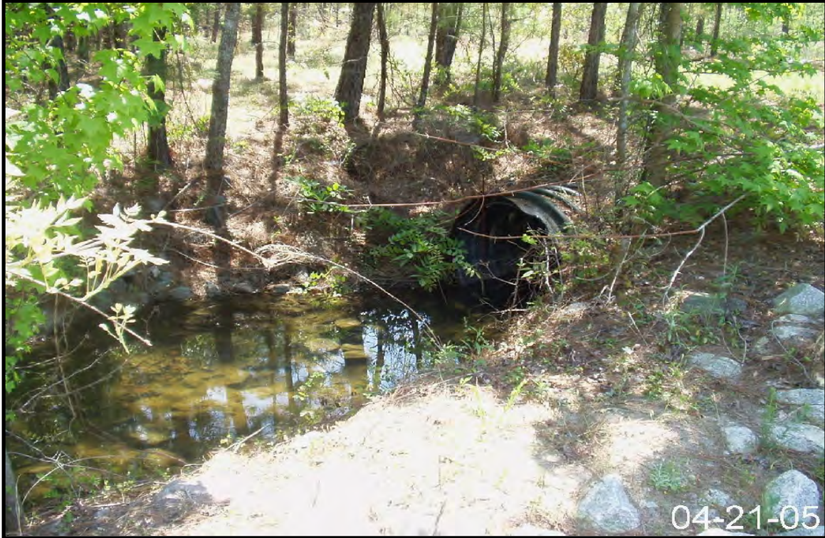
Figure 2-108. View of Stormwater Outfall N-16.
