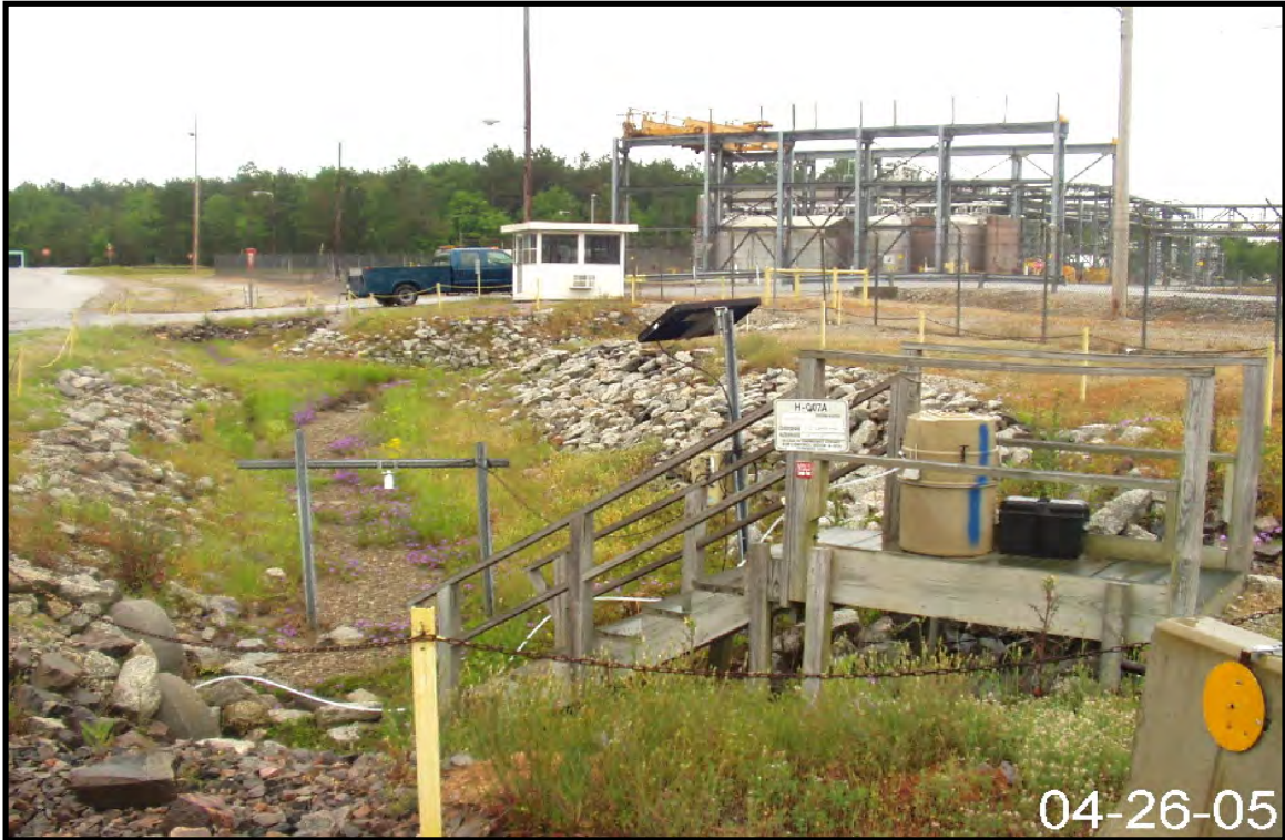
Figure 2-42. View of Stormwater Outfall H-7A.
