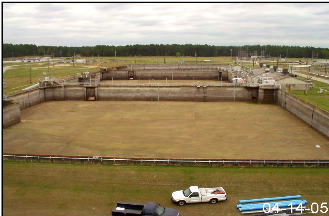
Figure 2-13. Representative View of Drainage Area for Stormwater Outfall C-04.
