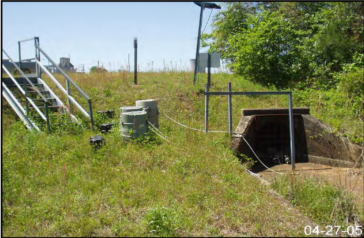
Figure 2-55. View of Stormwater Outfall K-02.
