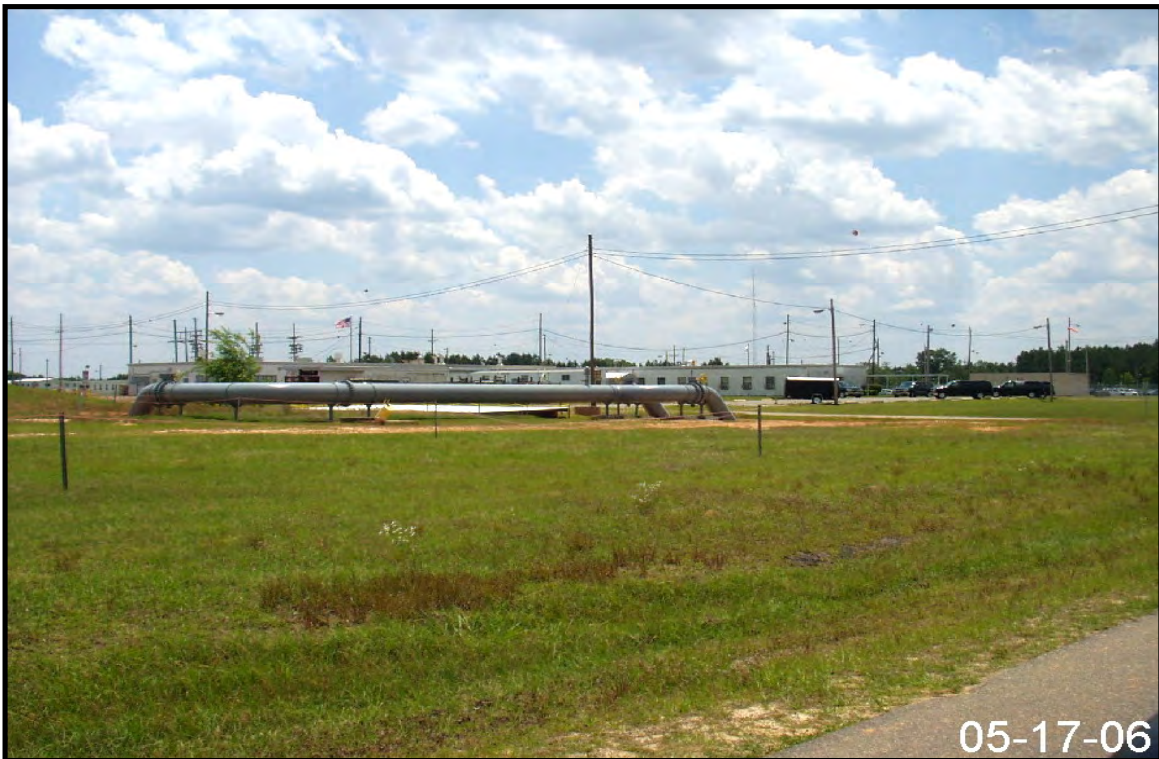
Figure 2-69. Representative View of Drainage Area for Stormwater Outfall L-13.
