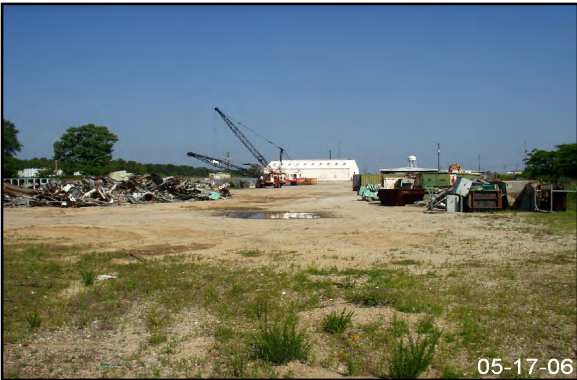
Figure 2-98. Representative View of Drainage Area for Stormwater Outfall N-12A.
