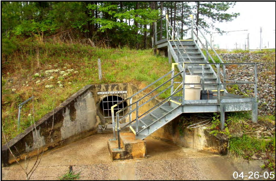
Figure 2-39. View of Stormwater Outfall H-06.
