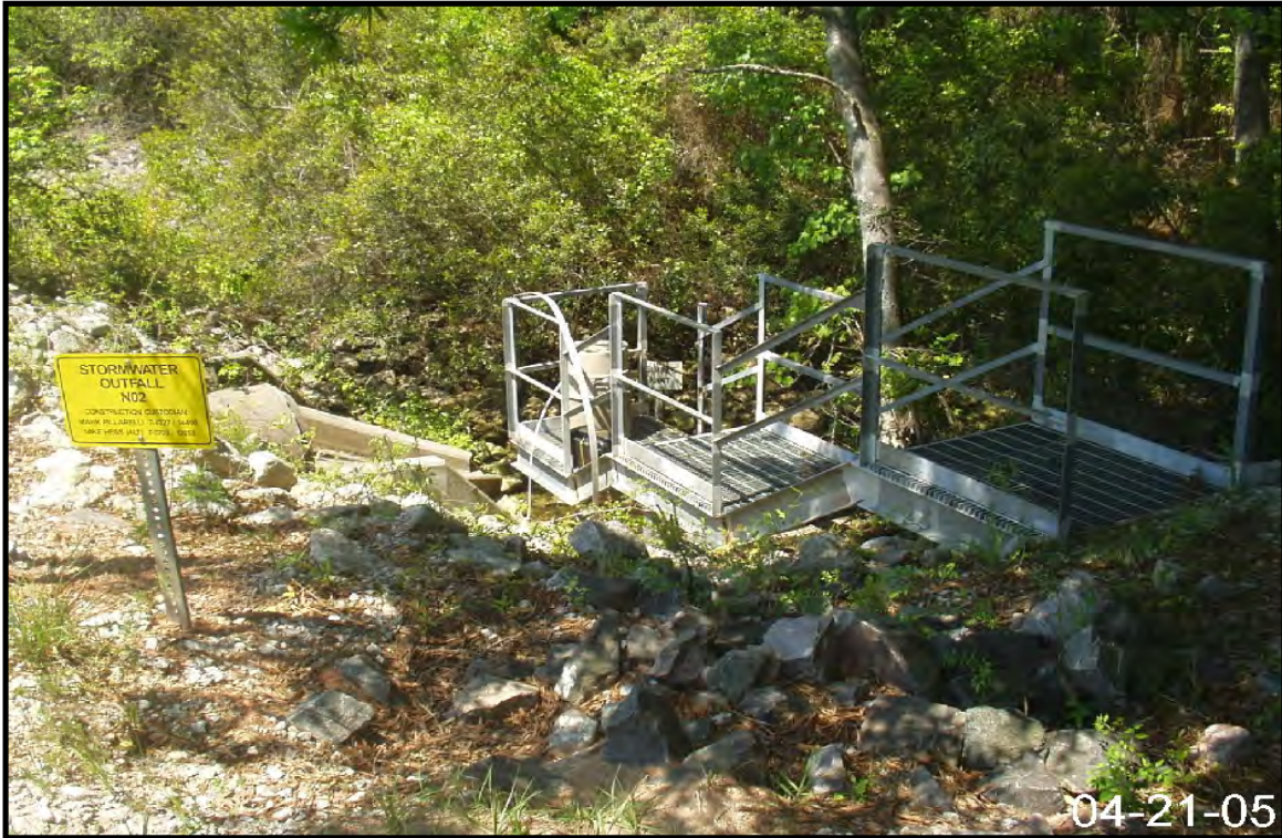
Figure 2-75. View of Stormwater Outfall N-02.
