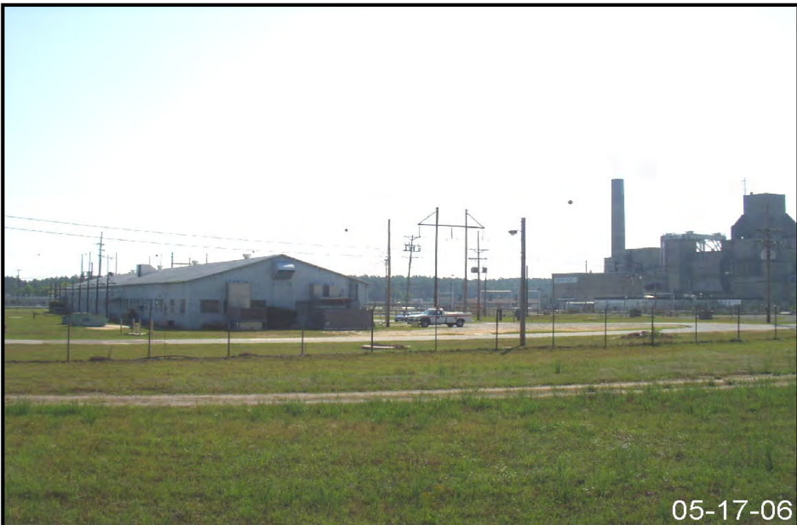
Figure 2-10. Representative View of Drainage Area for Stormwater Outfall C-01.
