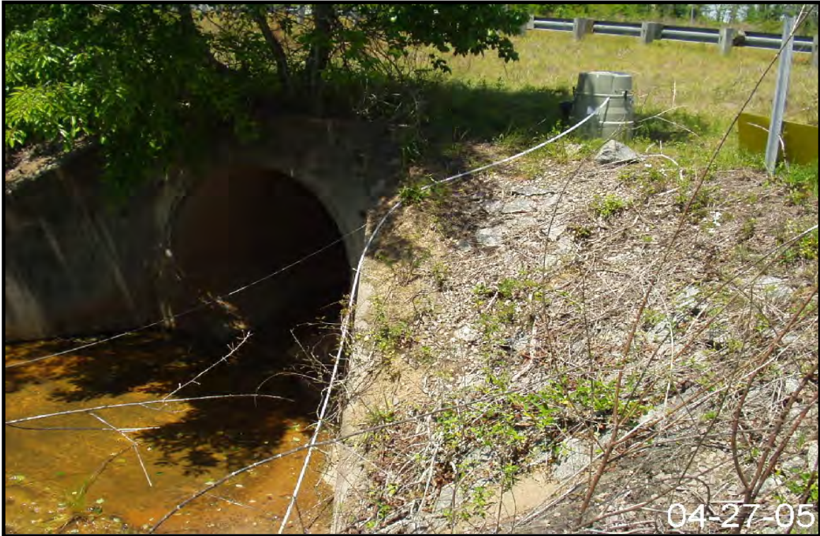
Figure 2-62. View of Stormwater Outfall L-03.
