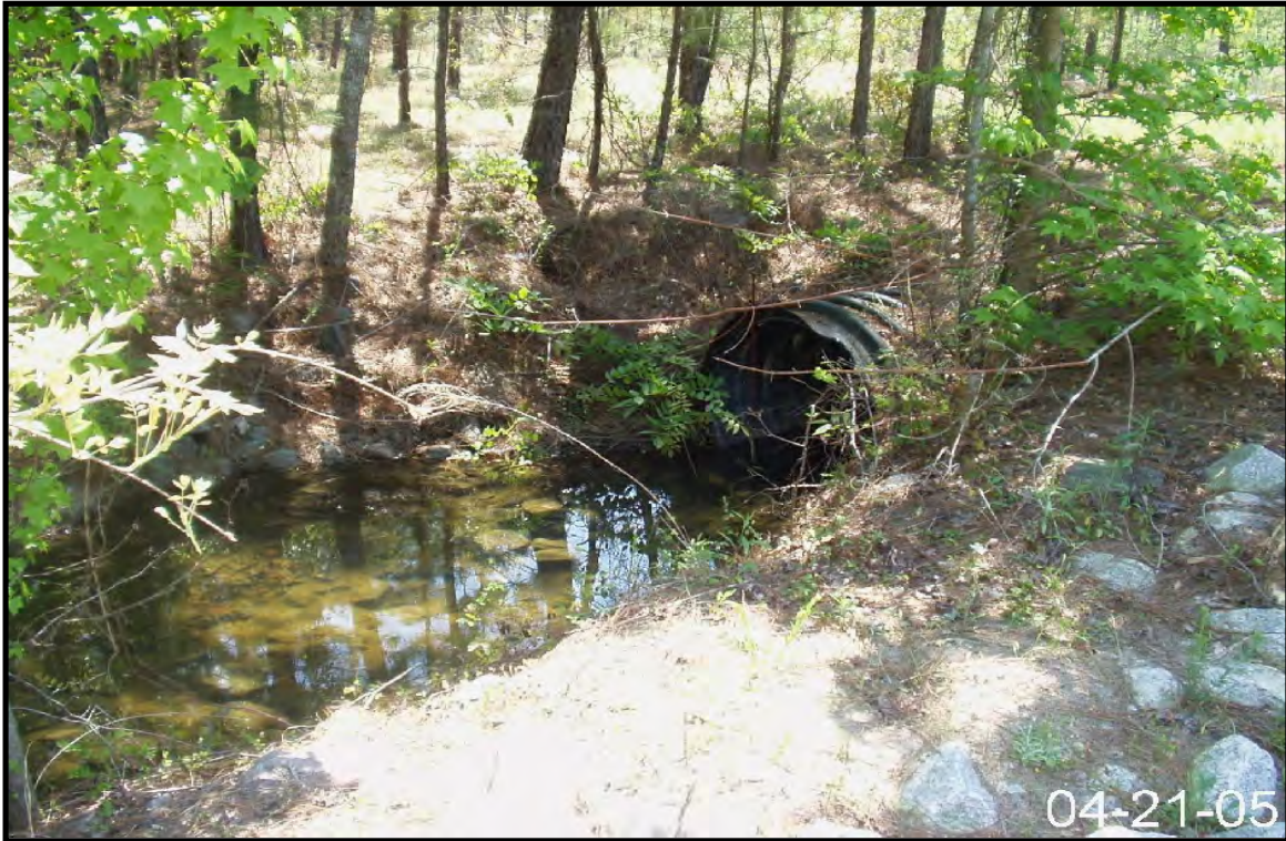
Figure 2-108. View of Stormwater Outfall N-16.
