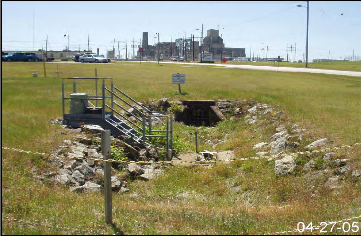
Figure 2-51. View of Stormwater Outfall K-01.
