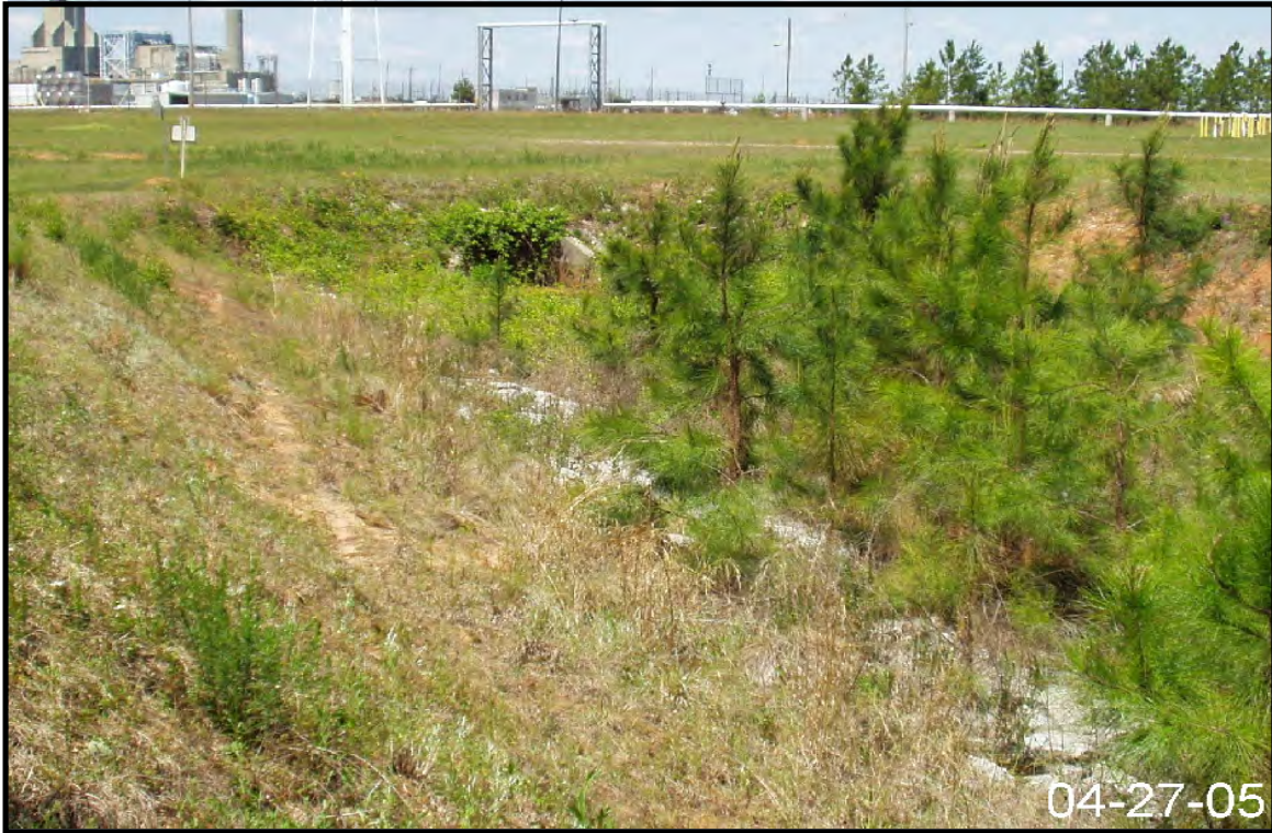
Figure 2-59. View of Stormwater Outfall K-04.
