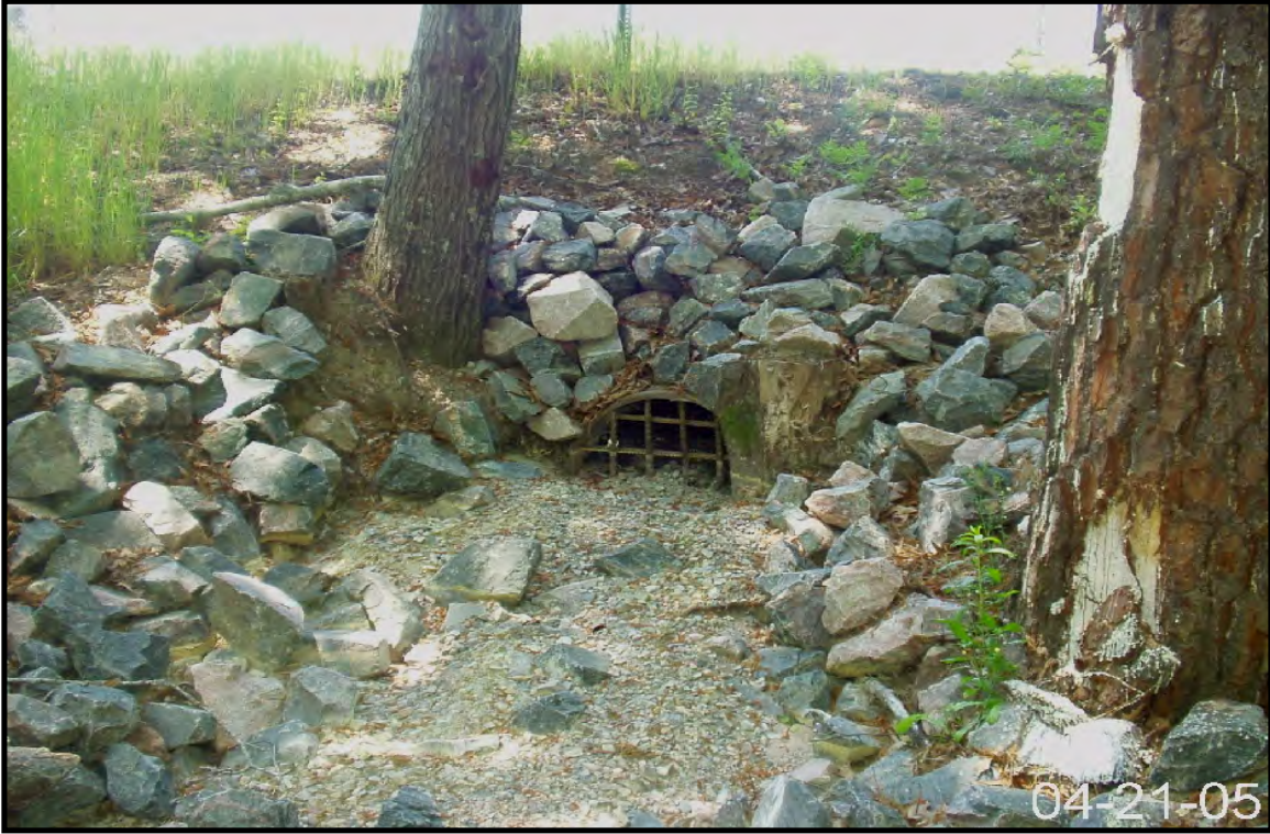
Figure 2-84. View of Stormwater Outfall N-05.
