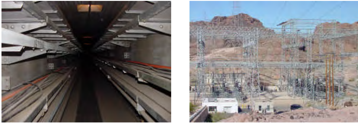
Figure 2-2. Photographs of Hoover Dam Control Tunnel with cabletrays which runs from the Hoover Power Plant to the Los Angeles Switchyard (shown on right).
