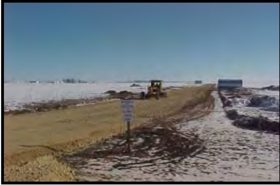
PREPARING THE ROADS
