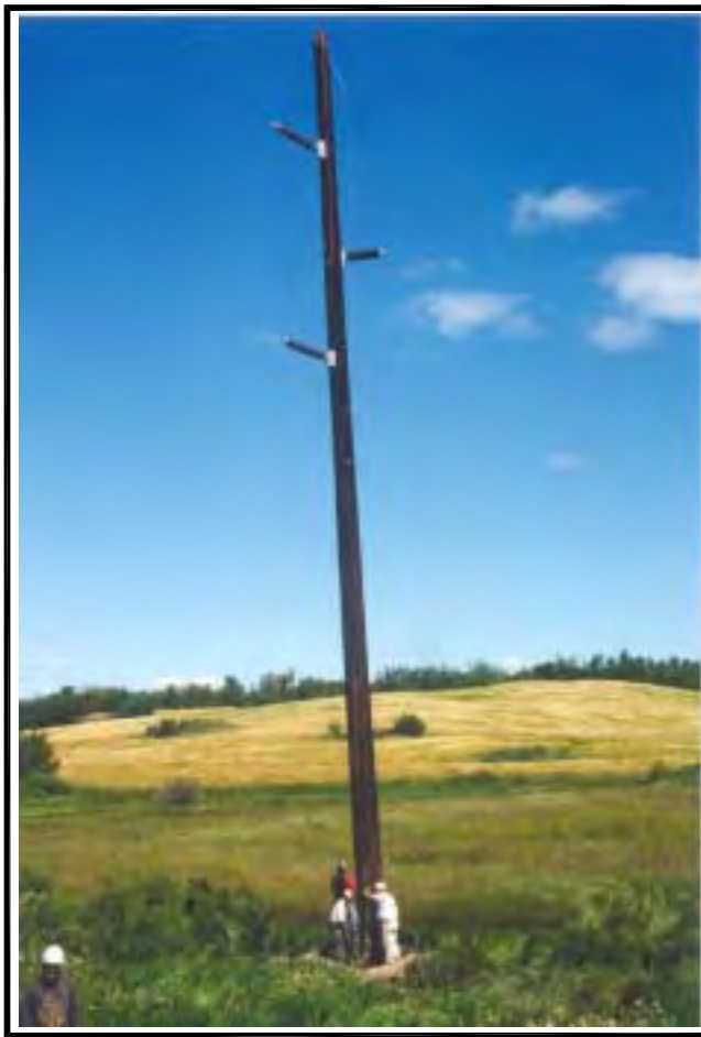
TYPICAL 115-KV WOODEN TRANSMISSION STRUCTURE
