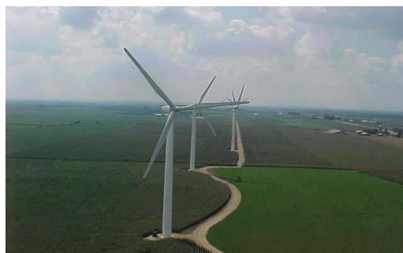
Typical Post-Construction Windfarm in an agricultural landscape.
