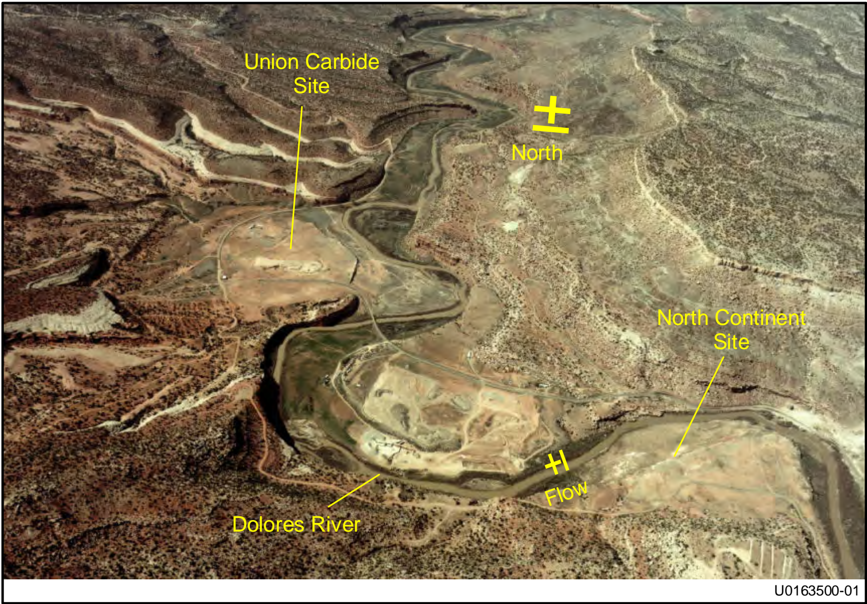
Figure 2. April 2001 Aerial Photograph of the Slick Rock Area
