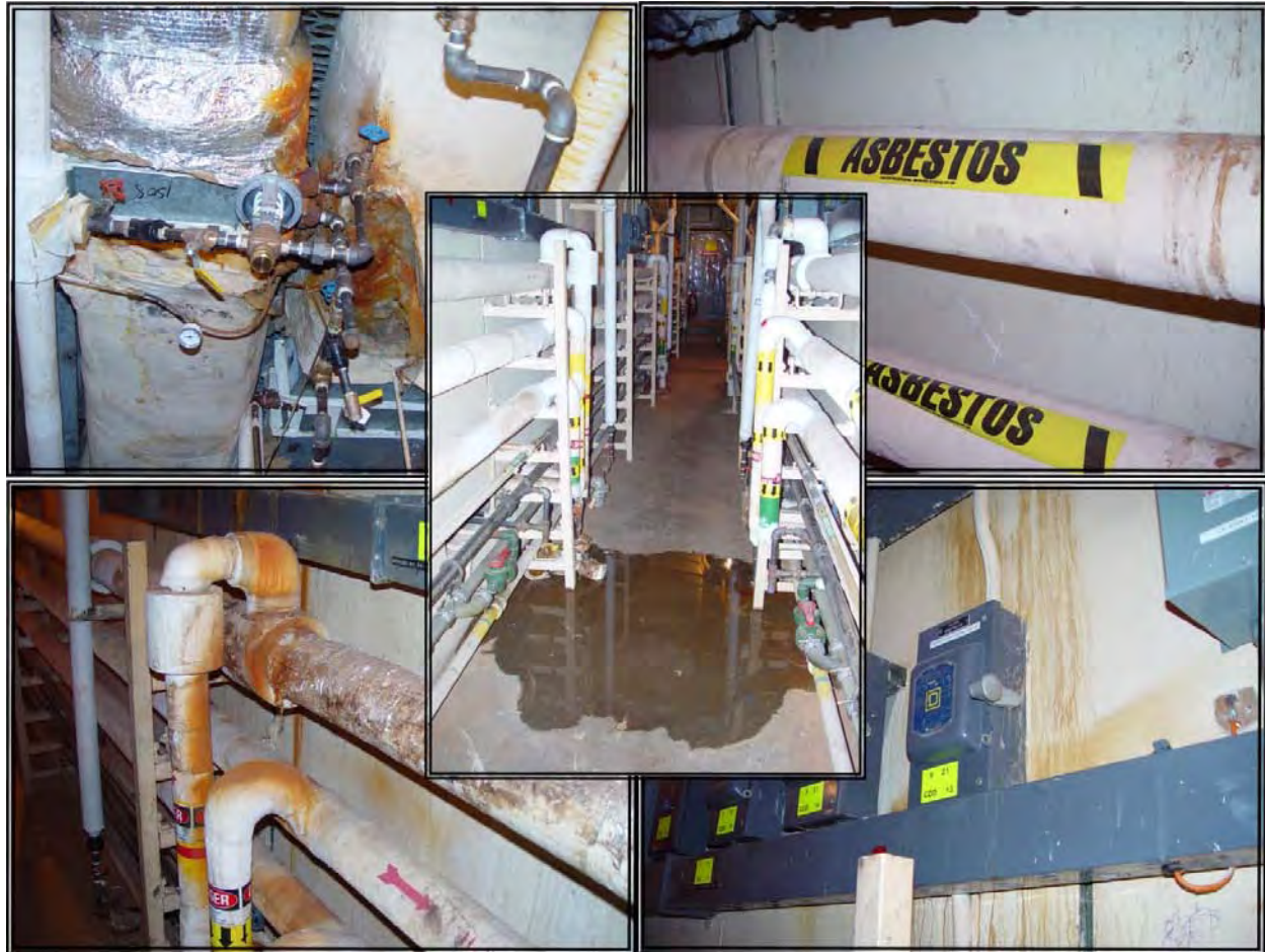
Photo 2. Maintenance problems at DX facilities.
