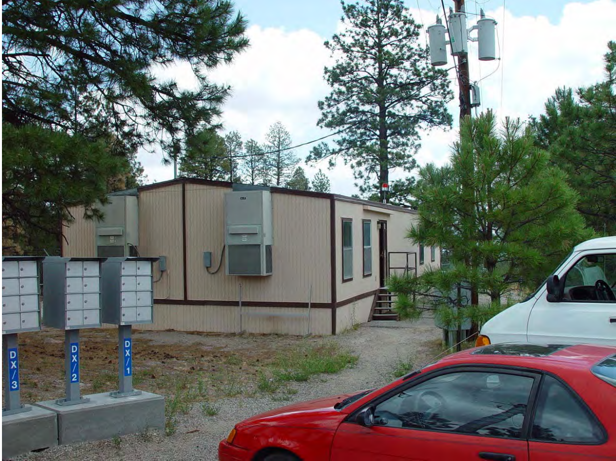
Photo 3. Transportable at TA-69 (Building 2).
