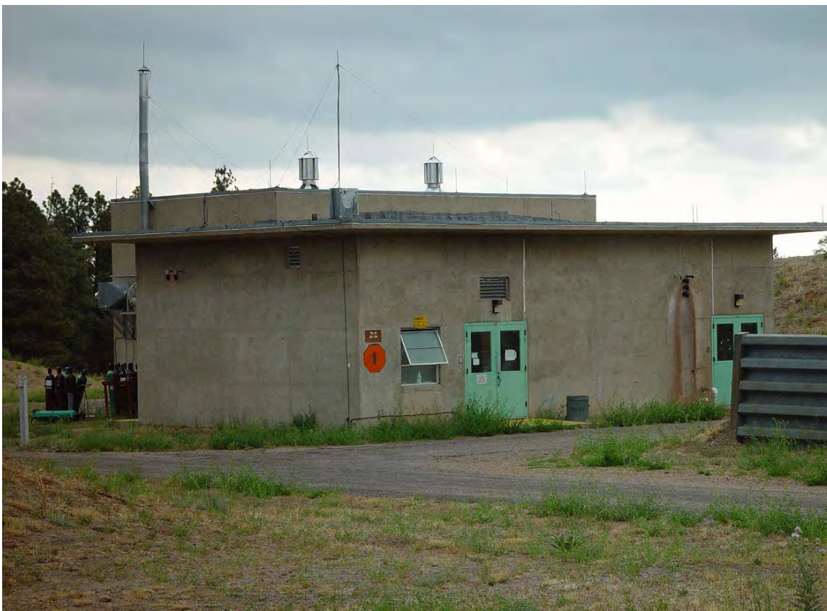
Photo 6. Typical energetic materials research building (TA-9 Building 34).
