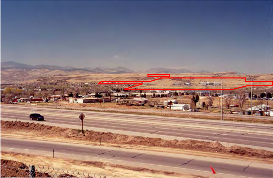
2. View of the STM Site from just south of Highway 6 (Sixth Avenue Service Road) looking north. The estimated future outline of long-term development is shown in red.
