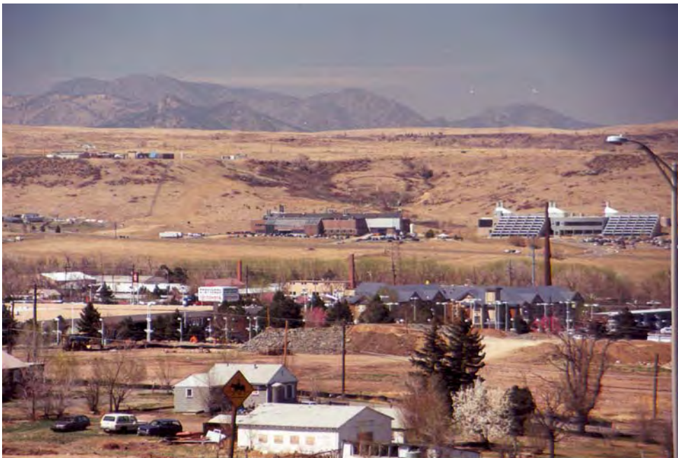
11. View of the mesa top facilities, FTLB and SERF from the 6 th Avenue frontage road (telephoto).
