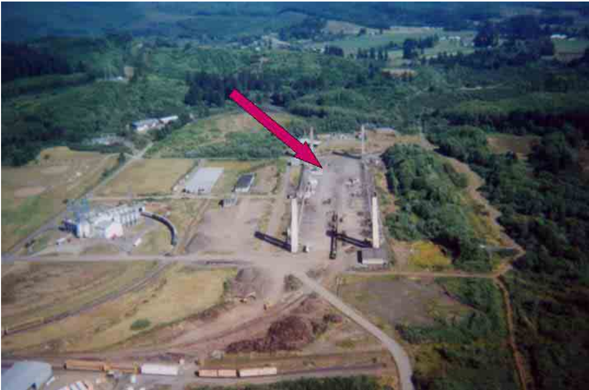
Figure 2. Aerial View of the 7.5-Acre Concrete Pad for the POTB Dairy Digester Site
