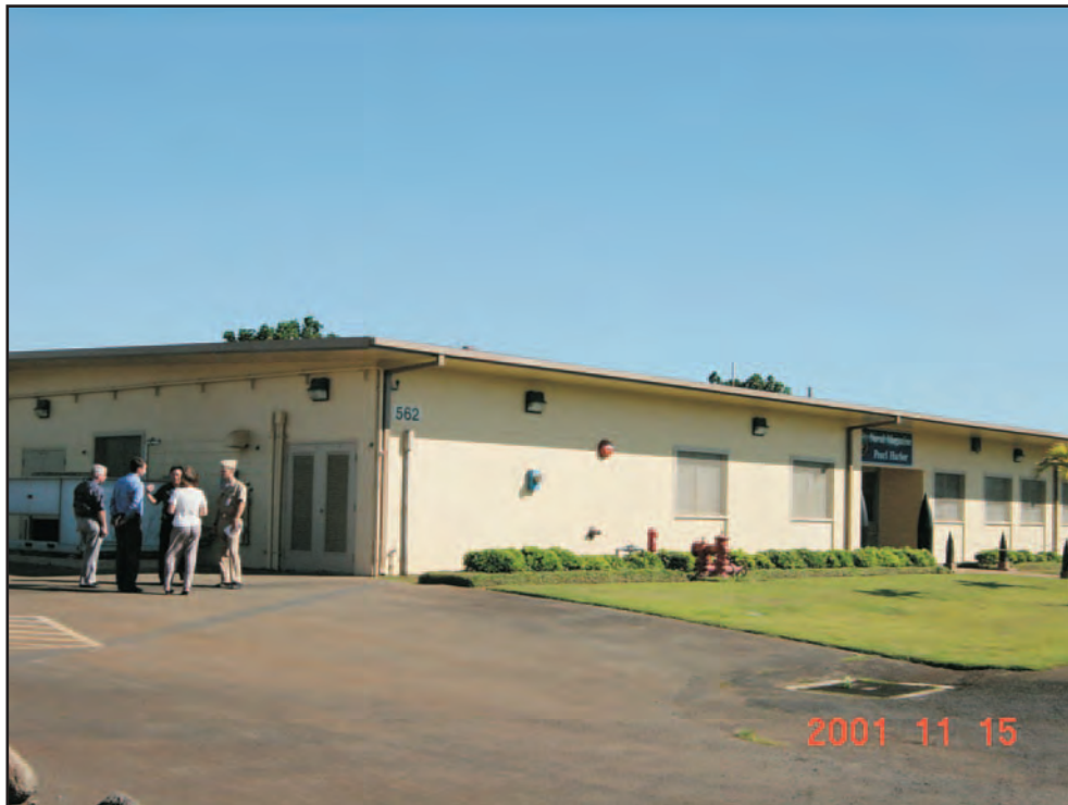
Building 562. Equipment shelter located inside double doors to the right of the group of people visible in the photograph.
