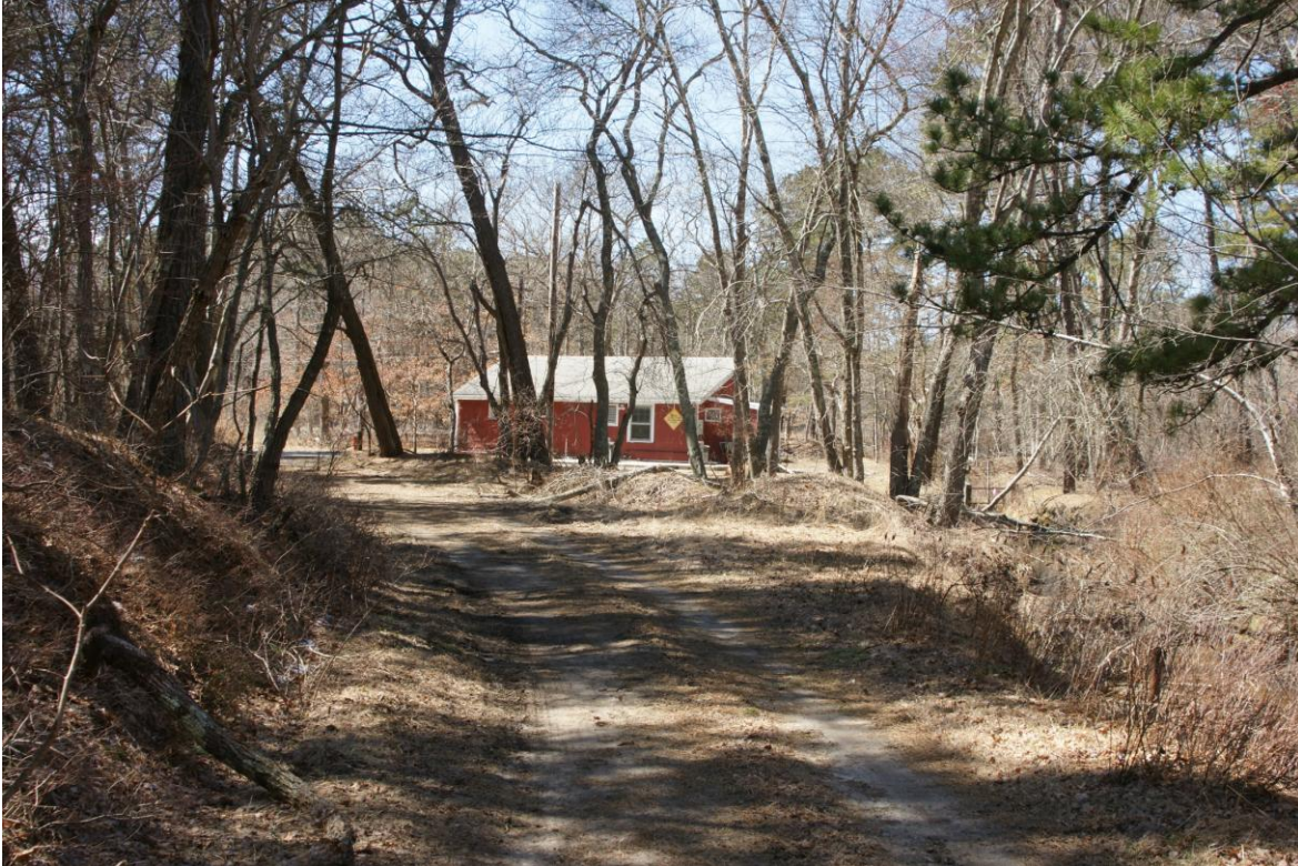
Figure 13: View from along the Peconic River looking west toward Bldg. 580. Bldg. 580 may be removed under Preferred and Enhanced Treatment alternatives.
