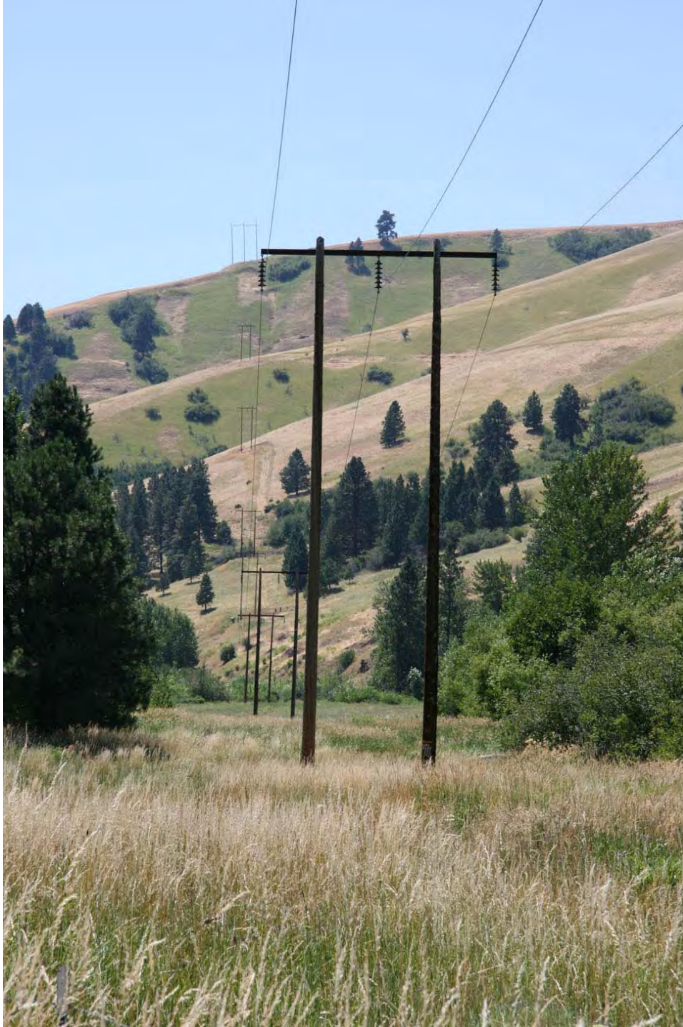
Figure 3-5. Structure 35/6 Looking Southwest
