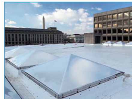
Cool roofs—as shown here on the DOE Headquarters building—use lighter-colored roofing surfaces or special coatings to reflect more of the sun's heat, helping to improve building efficiency, reduce cooling costs, and offset carbon emissions.
