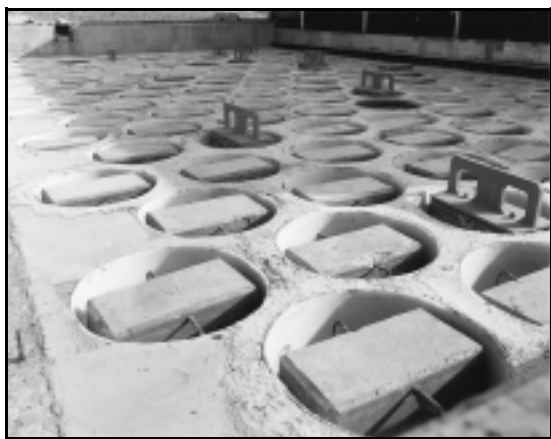
Intermediate Tritium Vault, Savannah River Site
