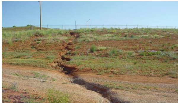
Figure 1: Erosion at the mill site
