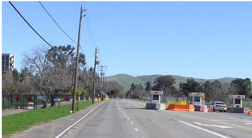
SOME OF THE NEWLY CONSTRUCTED SECURITY KIOSKS
