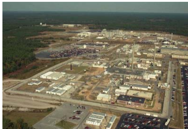
Aerial View of Tritium Facilities
