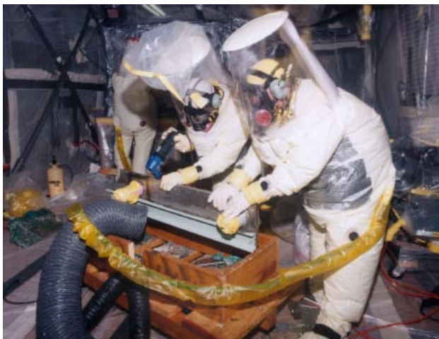
D&D Workers in Supplied Air Anti-Contamination Suits
