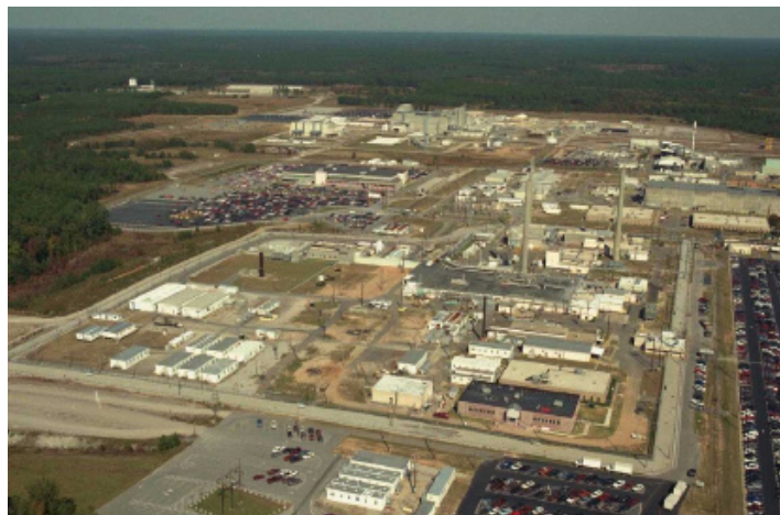
Aerial view of SRS
