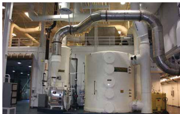
Decontamination and Waste Treatment Facility
