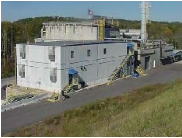
Aerial View of TWPC
