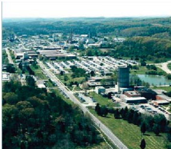
Aerial View of ORNL
