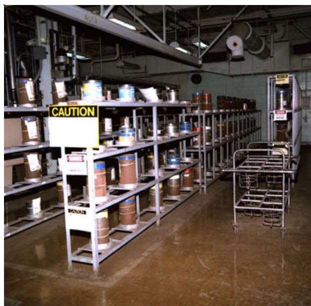
Storage Racks for Uranium Items
