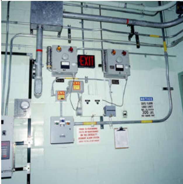
Criticality Accident Alarm System Equipment
