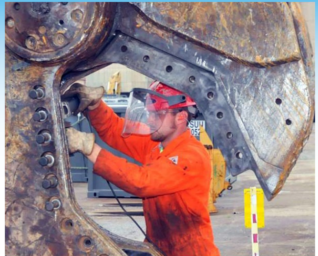
A worker removes bolts from shear blades used in decontamination and decommissioning work.
