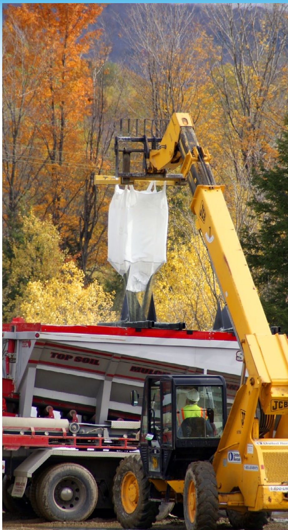
One-ton bags of zeolite are lifted over a truck called a “stone slinger” and cut open for placement in the trench.
