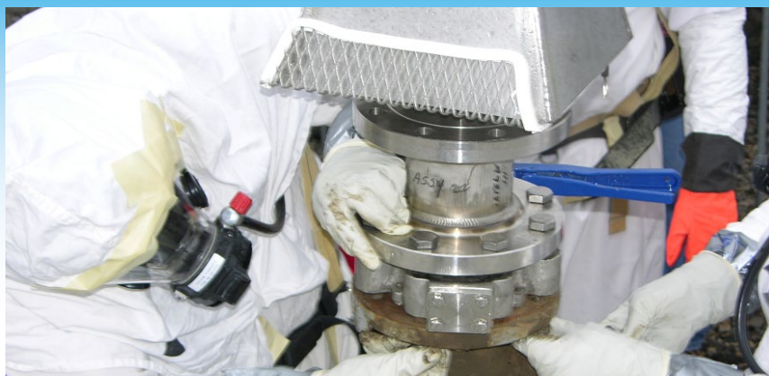
Recovery Act workers install one of the first of 113 filters for Hanford's single-shell tanks.
