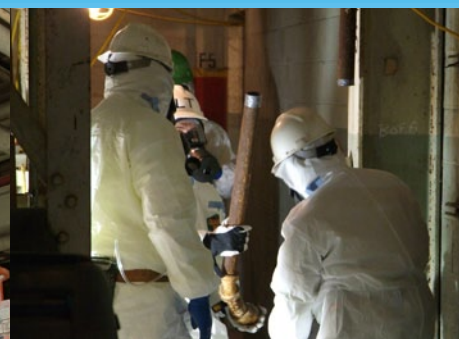
Recovery Act workers dismantle vacuum piping near the Slag Building of the old Metals Plant at the Paducah Site.
