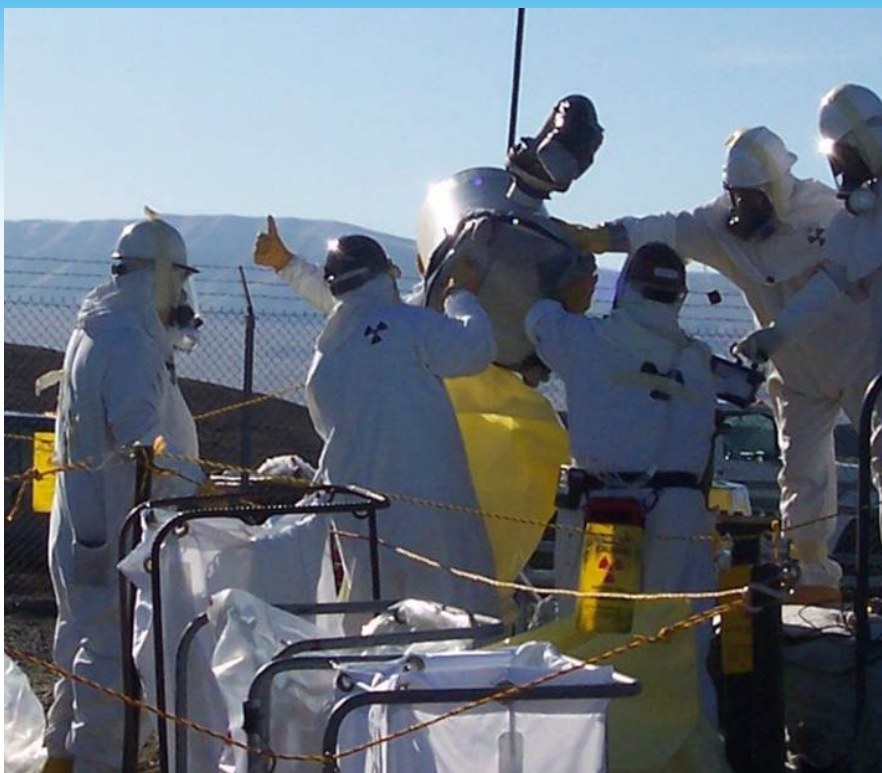
Workers change out the last of the obsolete filters. The replacement filters trap stray particles of contamination and reduce the risk of worker exposure.
