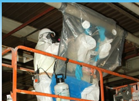
Recovery Act workers remove hazardous asbestos used for insulation throughout the old Metals Plant, one of two buildings scheduled for demolition at the Paducah Site.
