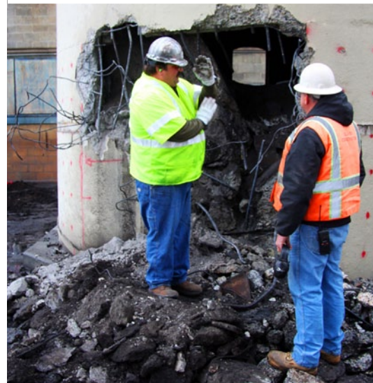
Above: Recovery Act workers removed a multi-layer security barrier at the Plutonium Finishing Plant after the last of nuclear material was removed from the facility in 2009. Workers removed razor wire fencing and concrete vehicle barriers and prepared inspection stations for demolition.
