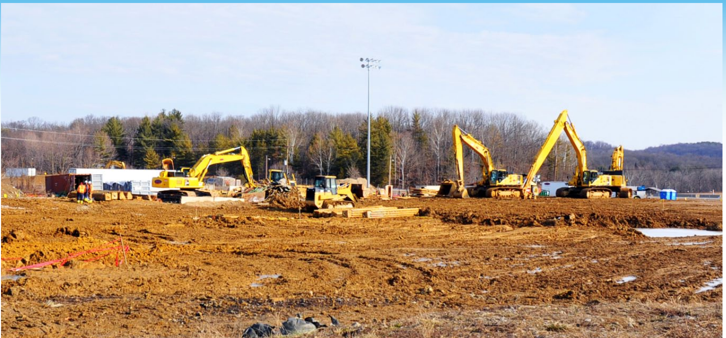
Final backfill operations are shown at the Portsmouth Site's X-701B Soils Treatment Project, which successfully reduced TCE levels by 95 percent.
