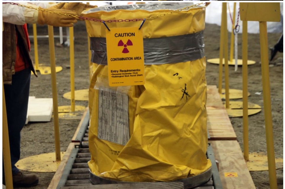
Photos above, a container of waste is excavated from an underground storage trench at the Hanford Site. Recovery Act workers place the container into protective covering and it is hoisted from the trench and staged adjacent to the trench for processing.
