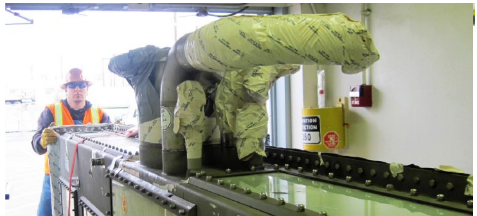
Top photo: Recovery Act workers remove a section of a glove box from the Plutonium Finishing Plant at the Hanford Site.
