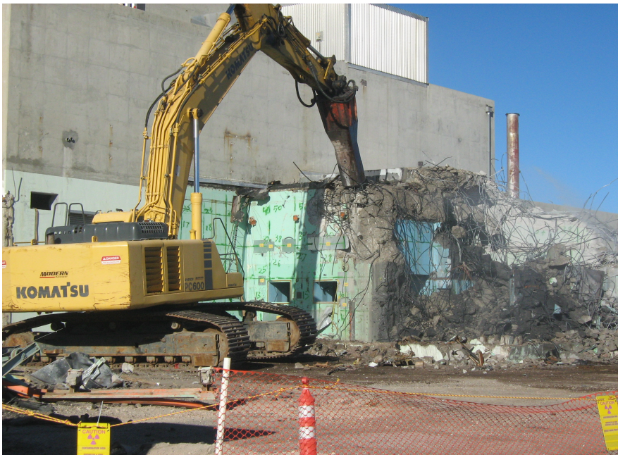
In the first phase of R-MAD's demolition, a hydraulic hammer was used to dismantle a section of the south block wall and roof.
