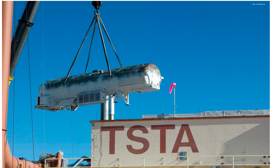
Nitrogen tank being taken off the roof of the TSTA building located on the TA-21 site. The tank was sent for metal recycling.
