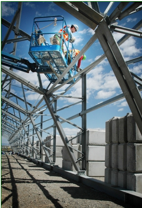
Workers prepare the steel structure of the ARP IV facility before the fabric skin can be installed.
