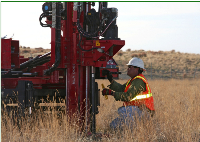
A North Wind employee prepares to install cone penetrometers into the trenches at the 618-10 Burial Ground.
