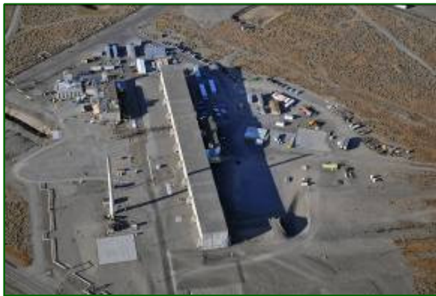
The exterior (above, left) and interior (above, right) of the 810-foot-long U Plant canyon on the Hanford site that is being readied for demolition. The canyon contains hundreds of pieces of radioactive, contaminated surplus or spare equipment that will be moved into 40 processor "hot" cells that are also part of the building.
