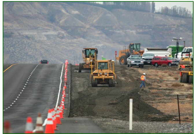
The 618-10 Burial Ground is located about five miles north of the city of Richland and right off the main Hanford site highway. Road crews are installing turn lanes on the four-lane divided highway to provide a safe entrance and exit for workers and equipment.
